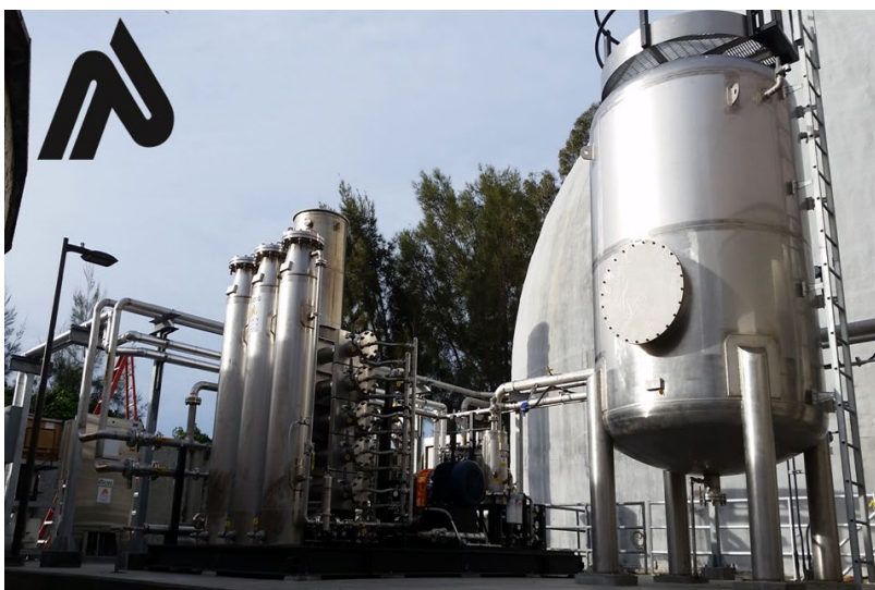
Figure 3-5. DG upgrading system at San Mateo WWTP (California) using Unison's BioCNG system Includes \text{H}_2\text{S} removal, moisture removal, compression, siloxane removal, and membrane separation.
