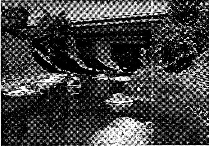
Photo 2 Interstate Hwy 101 crossing Santa Rosa Creek
