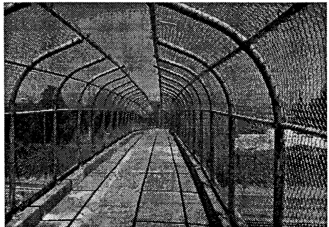
Photo 12 Existing pedestrian overpass on Hwy 101.
