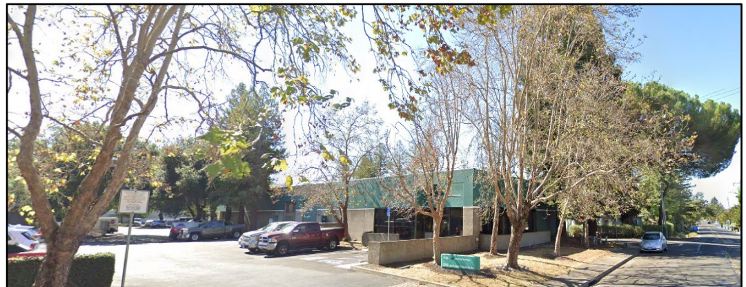
Building Entrance on Jennings Ave.
