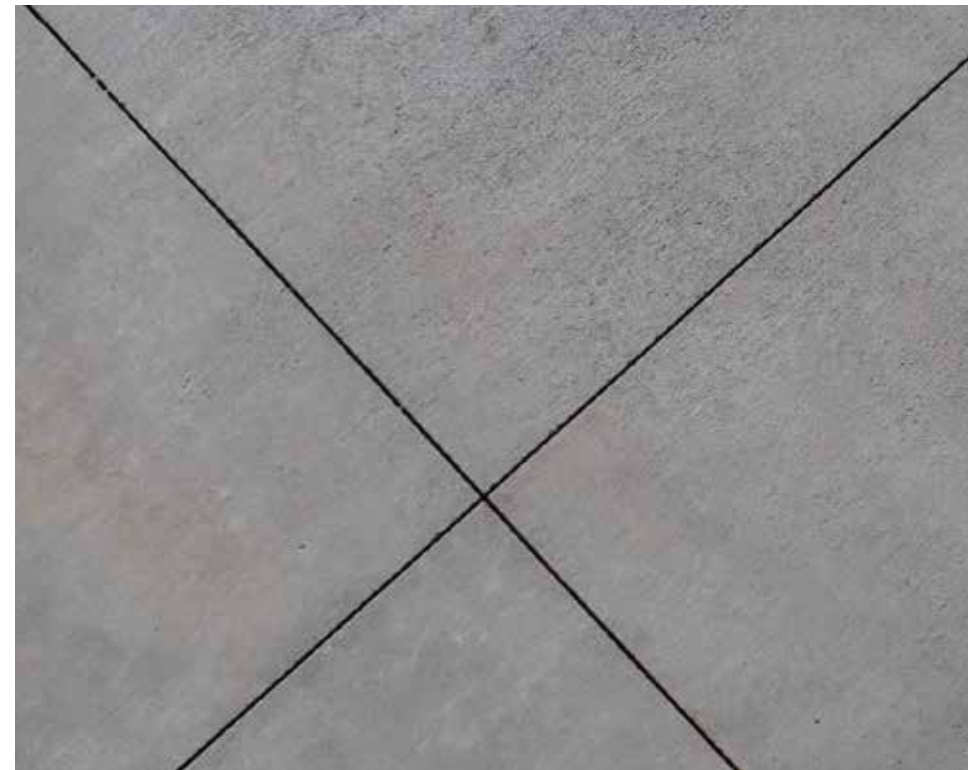
CONCRETE Saw Cut Joints
