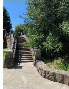
Prince Memorial Greenway Stairs to lower path from pedestrian bridge and central gathering space.
