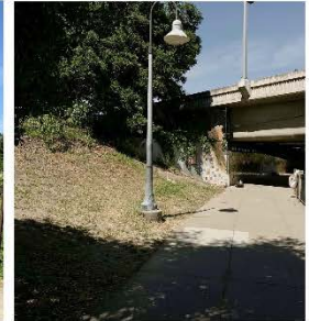
Prince Memorial Greenway Looking east. 101 Freeway overpass. Santa Rosa Creek to the right and down the slope.
