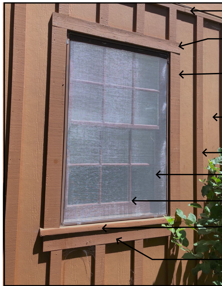
WINDOW/DOOR TRIM, SIDING DETAIL
