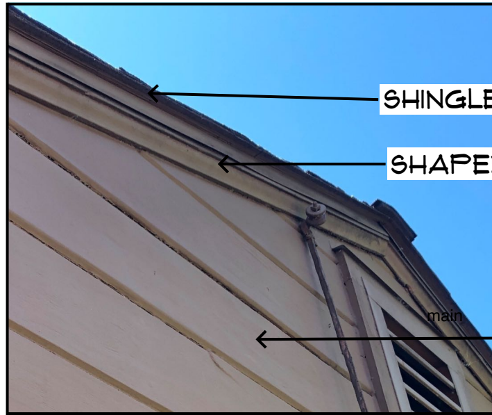
RAKE WALL DETAIL
