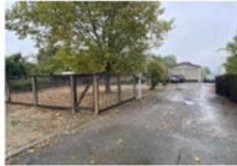
North (Front) Exterior – View From Street
