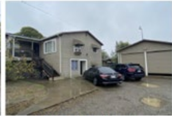
Northwest (Front) Exterior
