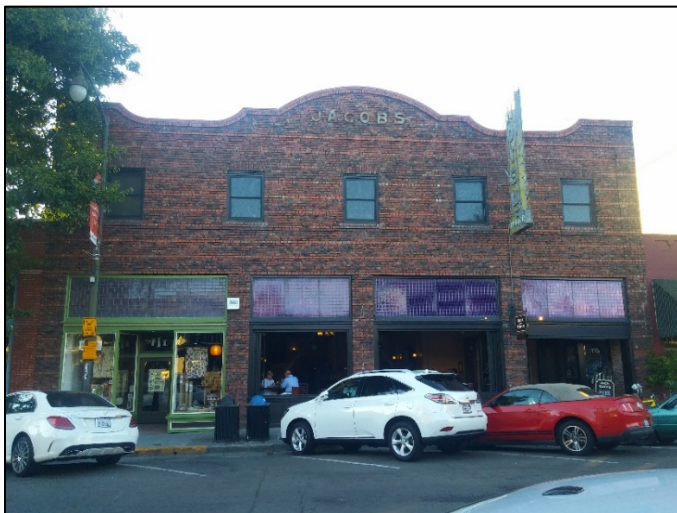
Jacobs Building south façade, 111-115 Fourth Street
