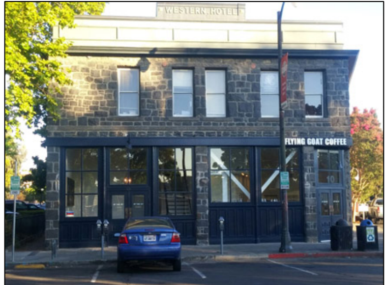
Western Hotel, north facade (note composition of elevation)
