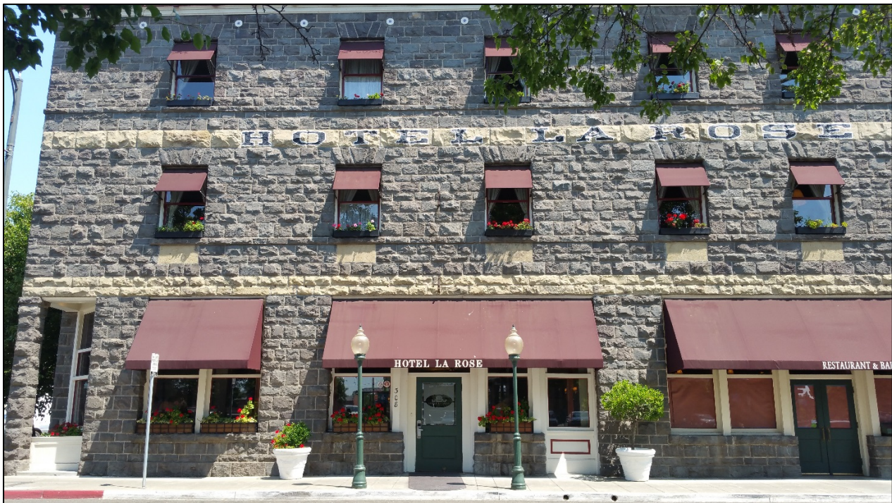
La Rose Hotel, western elevation (note façade composition, texture, door and window detailing)
