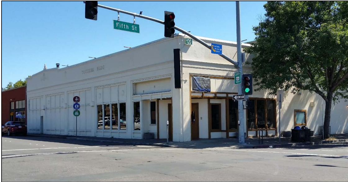
120 Fifth Street, view to southwest
