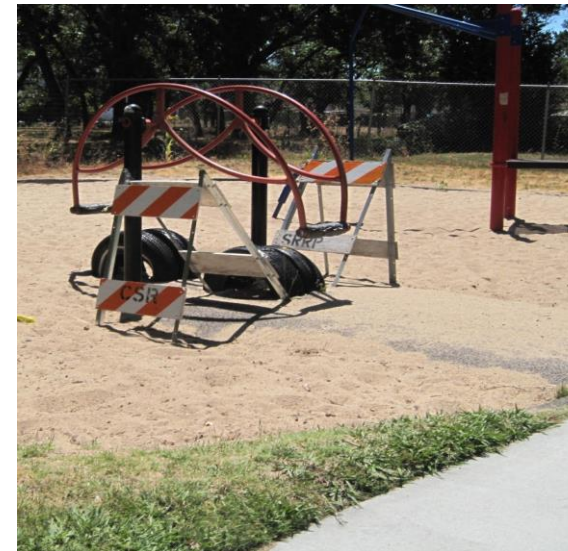
Broken and unsafe playground equipment
