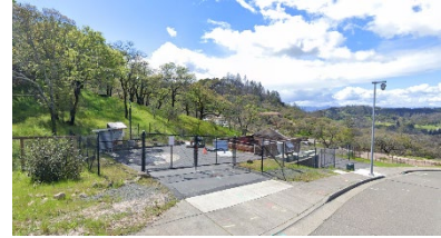
Skyfarm A Lift Station
