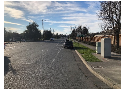
Pavement Preventative Maintenance Project – Petaluma Hill Road
