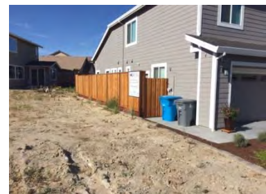
Figure 4 Wooden Fence Attached to Structure
