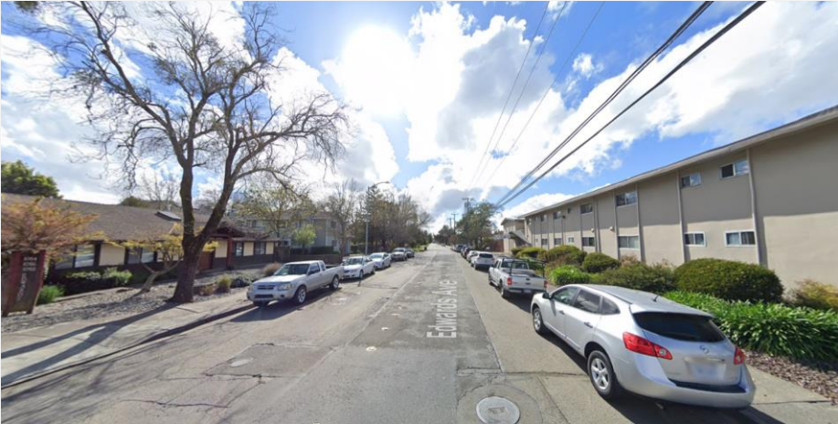
On Edwards Ave, View West
