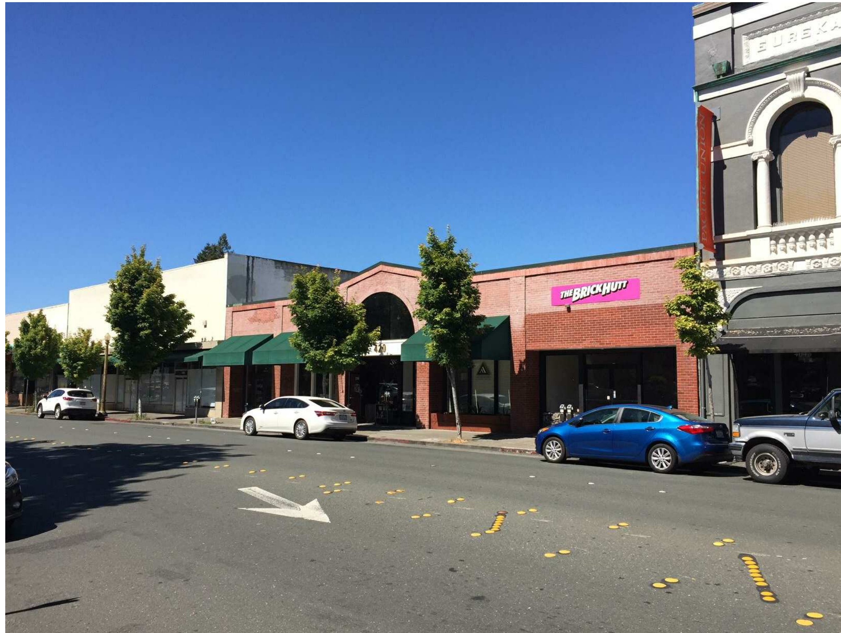
1. Mendocino Avenue, Looking north-west at 420 Mendocino
