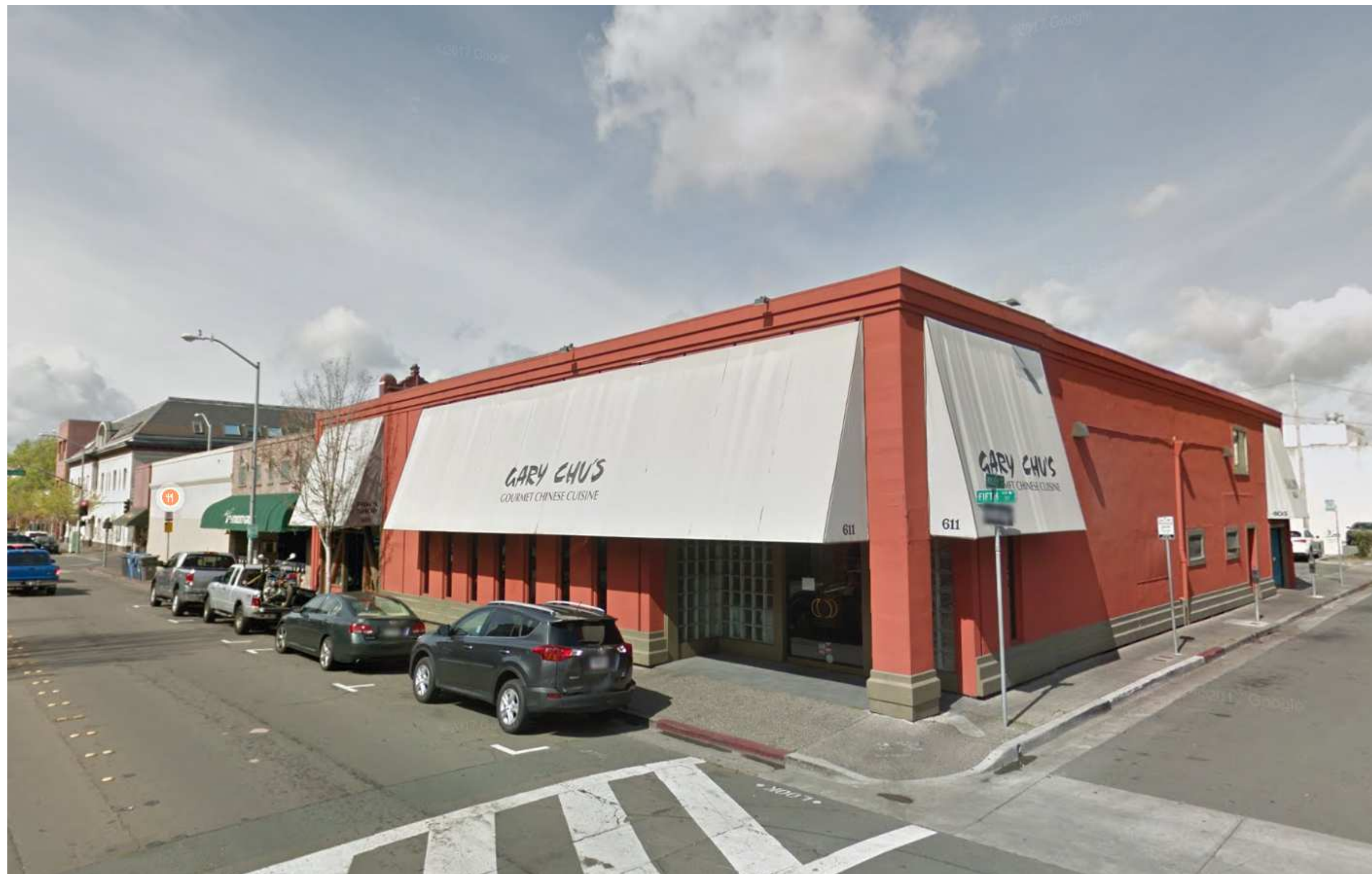
2. Fifth Street at Riley with existing building
