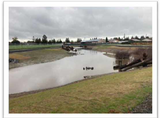
Figure 21 - Lower Colgan Creek Phase 2 after initial channel restoration, 2021
