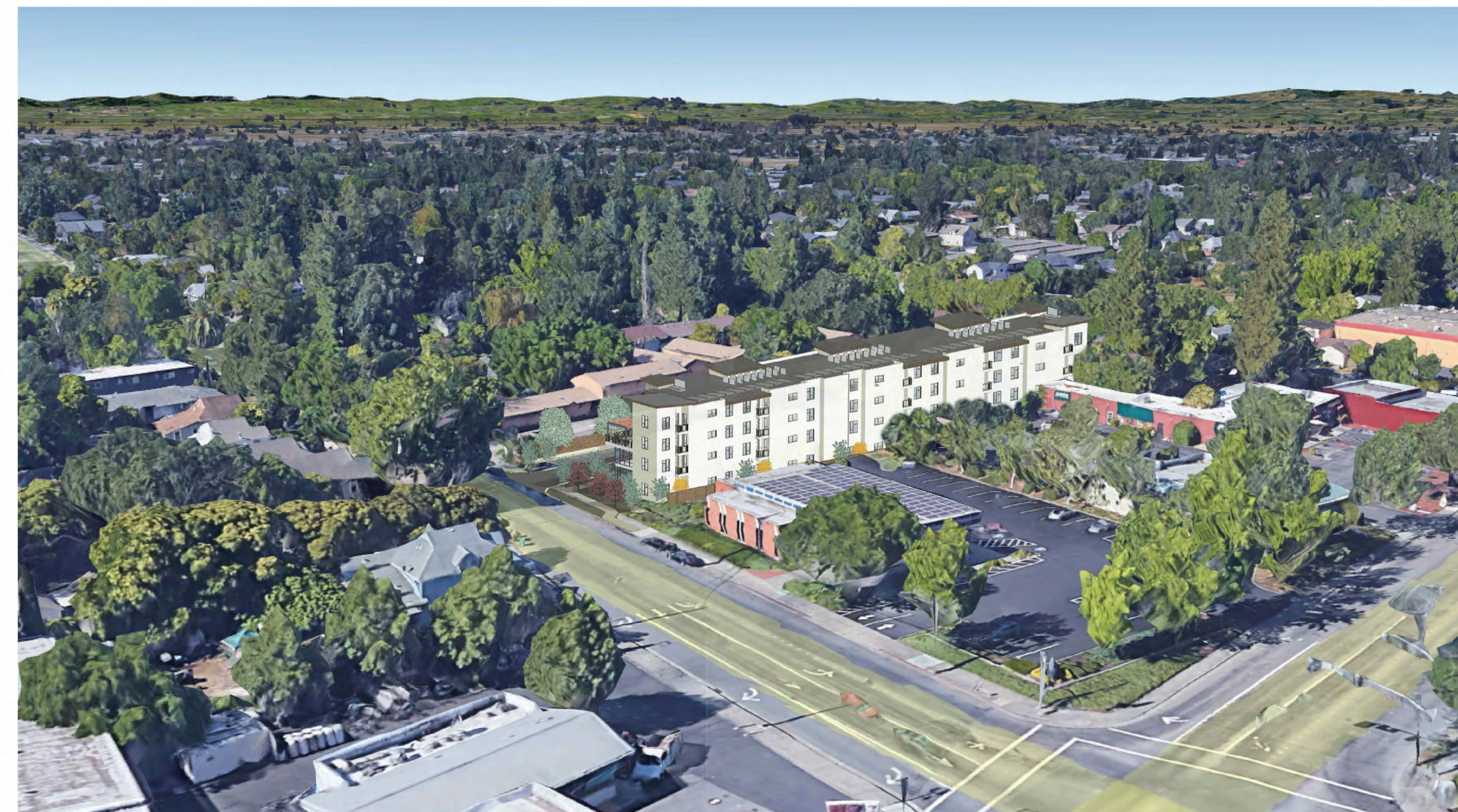
Aerial View from Northeast
