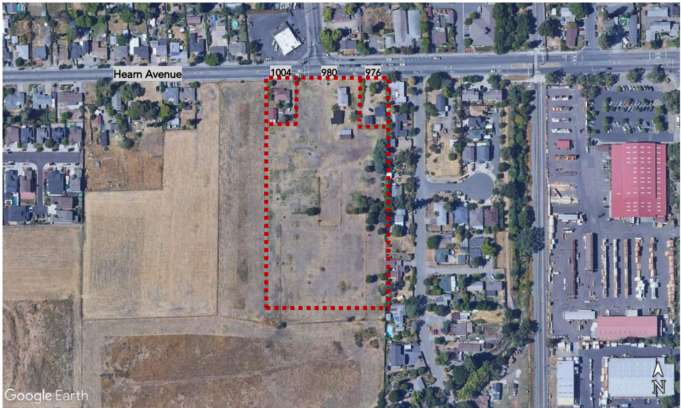
Figure 1. The subject properties on Hearn Avenue; the subject parcels outlined in red (Google Earth, imagery date June 2019).
