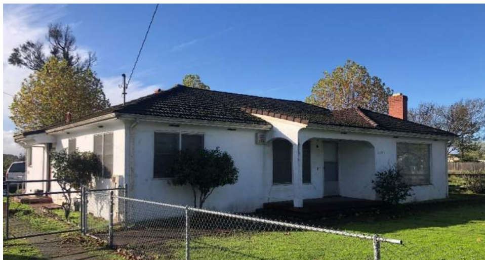
Figure 9. The front (north) and east façades of the house at 1004 Hearn Avenue.
