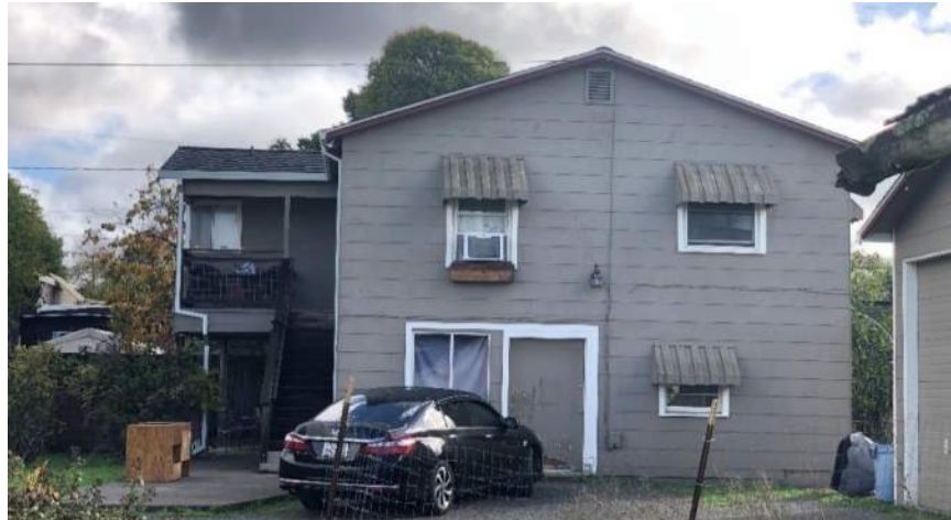
Figure 3. The west façade of the house at 976 Hearn Avenue.
