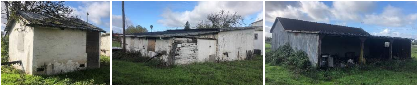
Figures 6, 7 and 8. The outbuildings to the south of the house.
