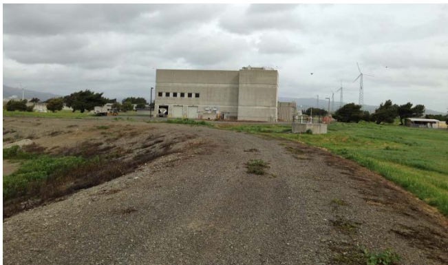
Dewatering Building and pipeline alignment to existing lagoons looking north
