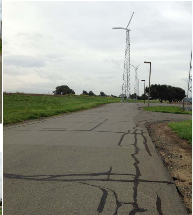
Pipeline alignment from Digesters to Dewatering Building looking south
