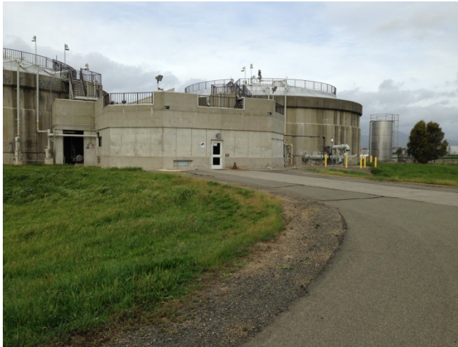
Digesters and north end of pipeline alignment looking northwest
