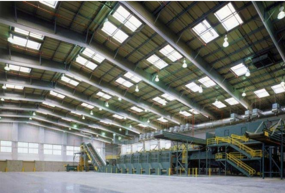
Enclosed Receiving Facility
