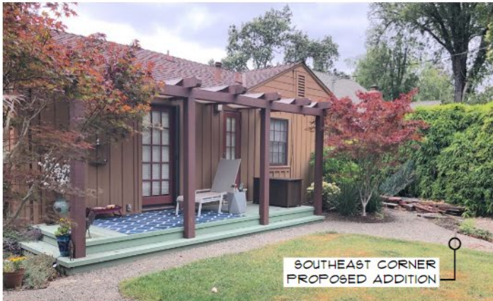
REAR YARD : VIEW LOOKING NORTHWEST
