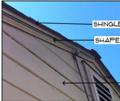
RAKE WALL DETAIL
