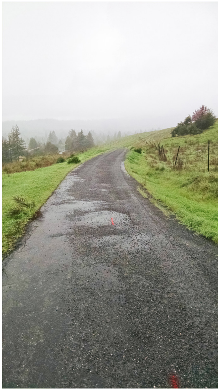
A: Existing access road looking west.
