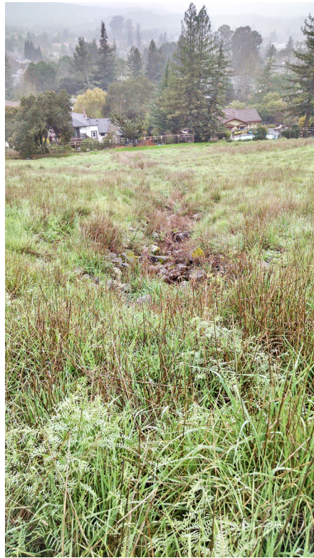
B: Existing rock slope protection downslope of access road.
