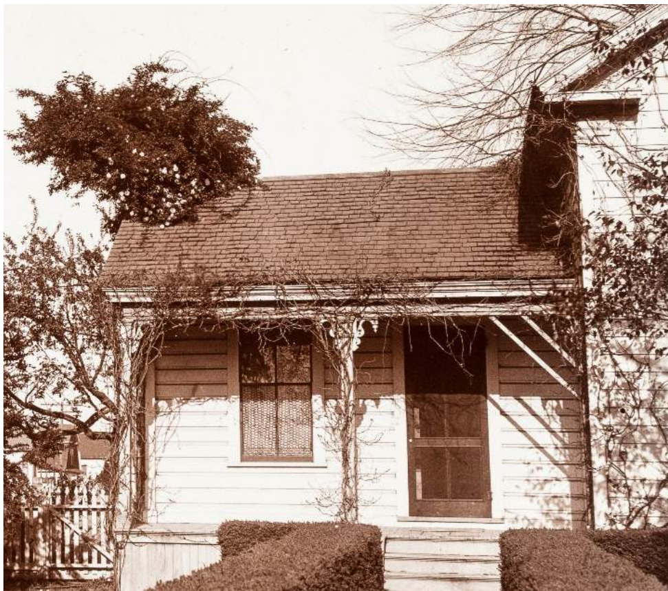
Image courtesy of the Luther Burbank Home & Gardens Association. c.1890. Only part of the original photograph is shown. Note wood shingle roof and lack of gutters or downspouts.
