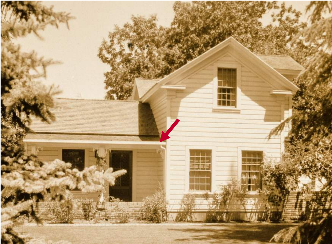
Image courtesy of the City of Santa Rosa and the Luther Burbank Home & Gardens Association c.1930. Only part of the original photograph is shown. Note wood shingle roof and new gutter and down spout at the porch (identified with the red arrow).
