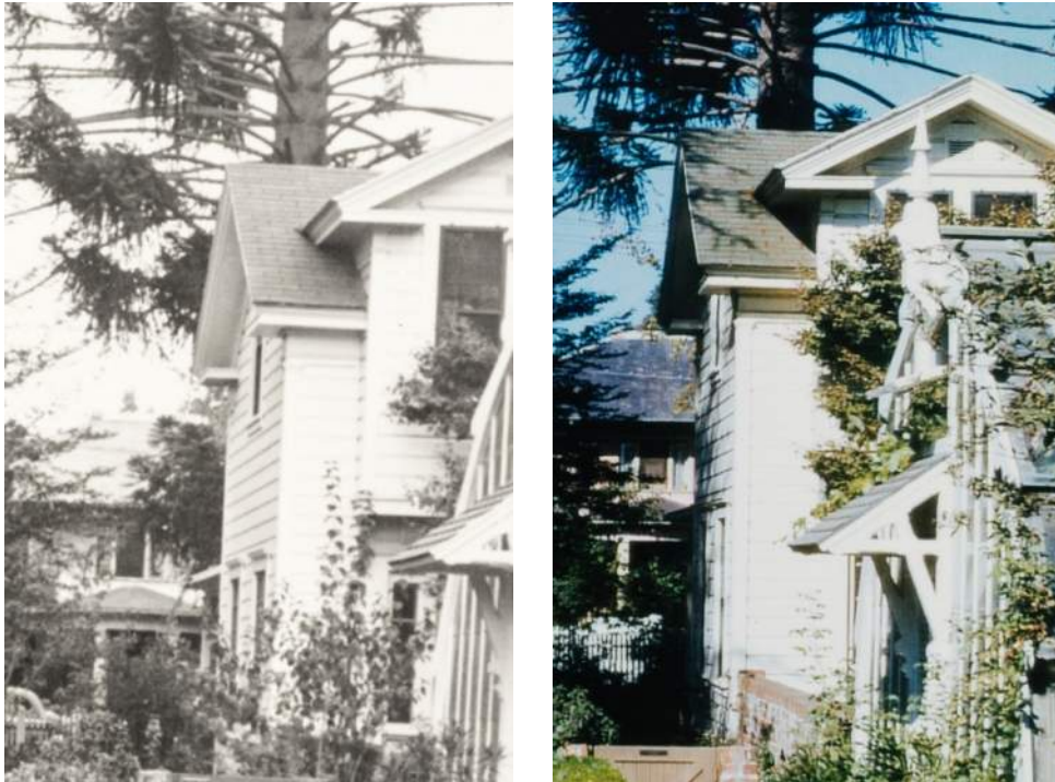
Images courtesy of the City of Santa Rosa and the Luther Burbank Home & Gardens Association. c.1940 (left) and c.1950 (right). Only part of the original photograph is shown. Note asphalt shingle roofing.
