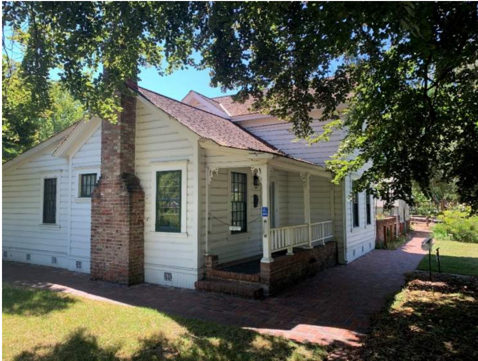
Current image of west elevation of Main House. Another alteration to the drainage system is that the existing wood box gutter integral to the cornice has been shingled over at this location.
