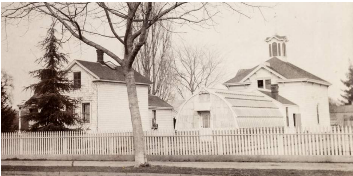
Image courtesy of the Luther Burbank Home & Gardens Association. c.1890. Only part of the original photograph is shown. Note wood shingle roof on Carriage House.
