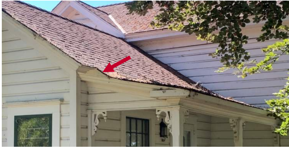
Current image of porch roof on west elevation of Main House.
