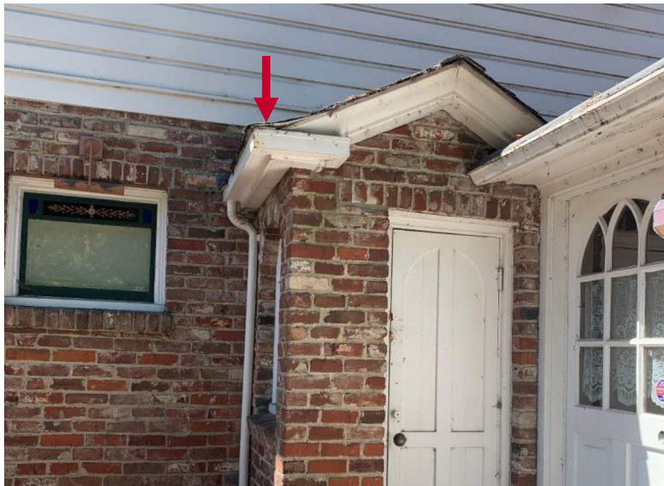
Current image of rear (north) elevation of Main House. An alteration to the drainage system is that the existing wood box gutter integral to the cornice has been shingled over at this location.
