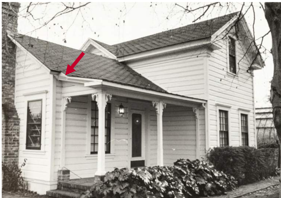
Image courtesy of the Western Sonoma County Historical Society Collection c.1940. Rolled asphalt roofing has been applied to the roof of the Main House. Note connection between the main roof and the porch roof (red arrow).
