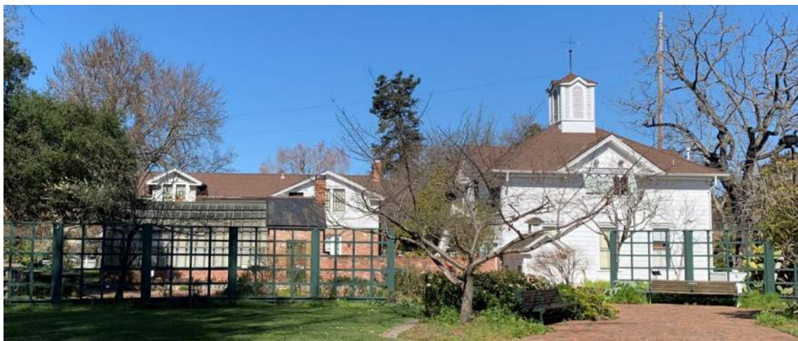
Current image of south elevation of Carriage House. Note existing red-brown color of the asphalt roofing.
