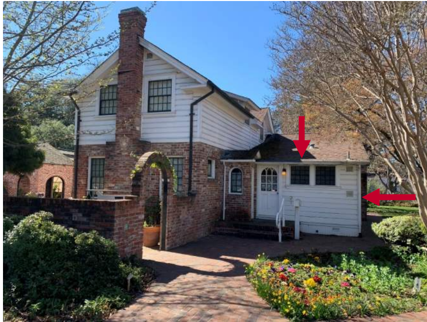
Current image of rear (east) elevation of Main House. Note the existing asphalt roofing is a red-brown color. One alteration to the gutters and downspouts is the installation of a new gutter and downspout on the east elevation (red arrows). This newer gutter and downspout replaced the existing wood box gutter integral to the cornice that was shingled over and abandoned at this location.
