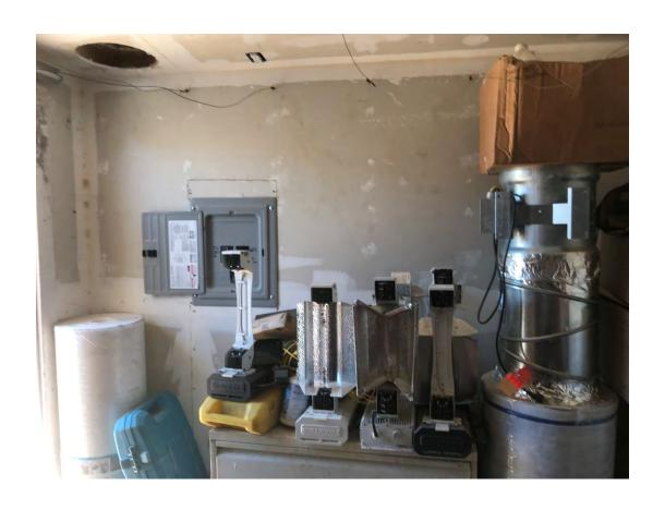
2620 Iroquois St wind turbine and penetration of sheetrock Possible issue with fire rating / electrical
