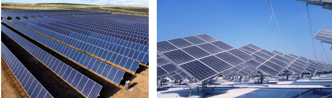
Figure B-2: Single-Axis and Dual-Axis Tracking Systems
