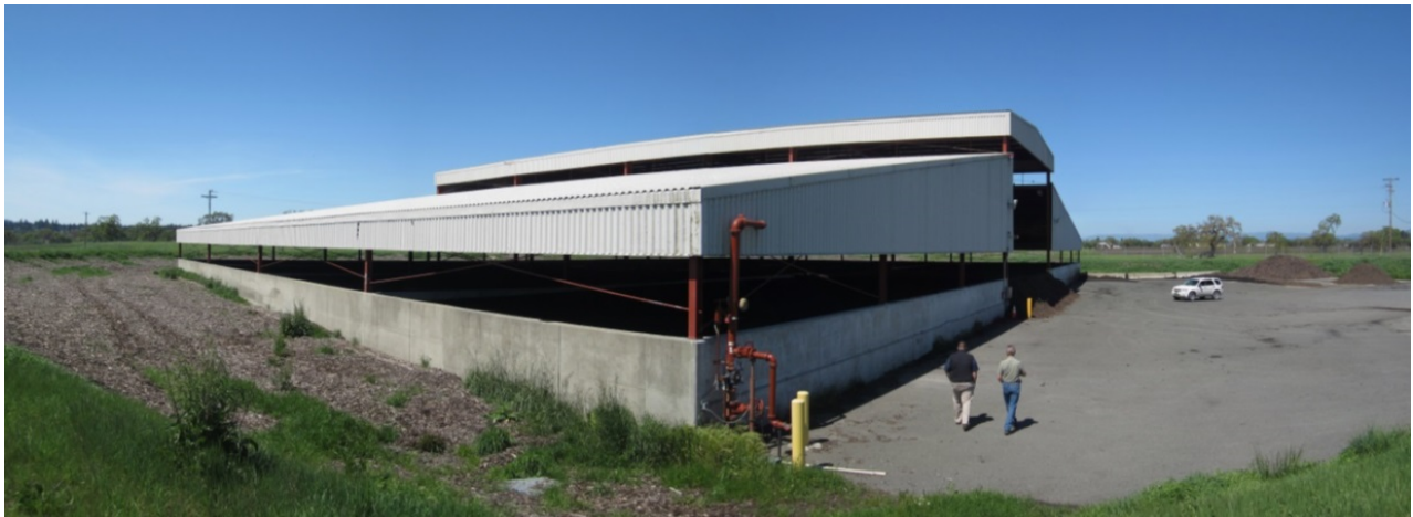
Figure 2-7: Alpha Farm Biosolids Storage Building
