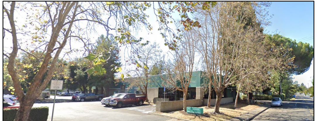
Building Entrance on Jennings Ave.
