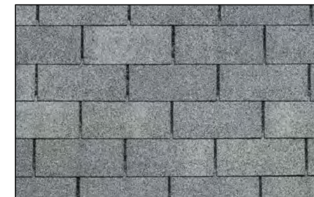
GRAY ASPHALT SHINGLE ROOF
