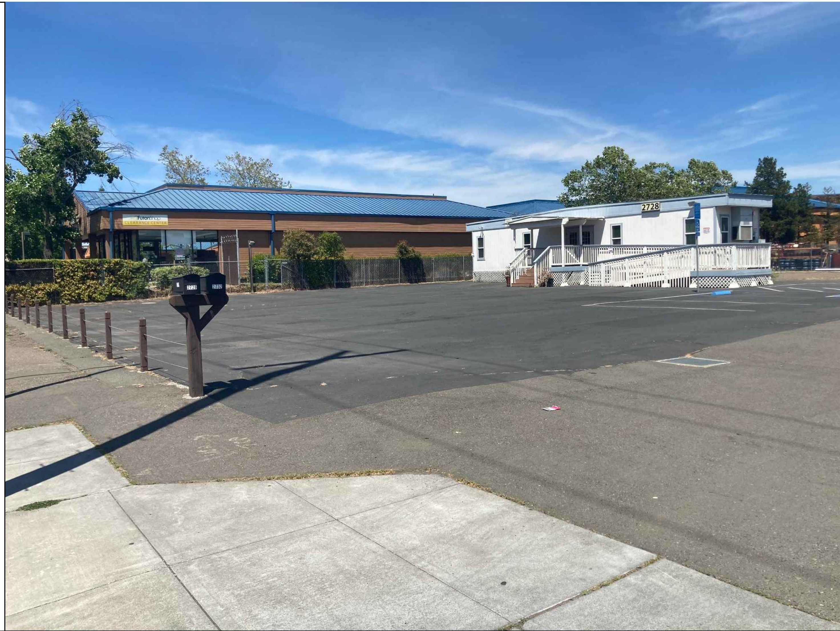
VIEW FROM SW CORNER OF LOT
