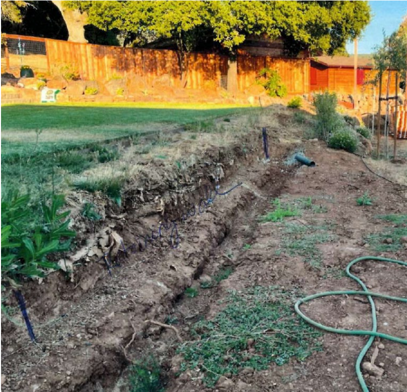
Grade change between 5022 Boulder and 5026 Boulder, from the backyard of 5022 Boulder
