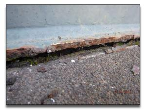
**Photo No. 5** – Annular ring wall with moss growing under tank.
