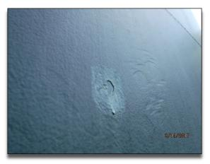
**Photo No. 18 –** Exterior coating repair of R-9A likely from rock damage.
