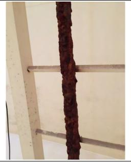
Photo 2-4. Interior Ladder Saf-T-Climb with Corrosion Product on the Surface
