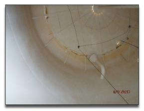
**Photo No. 4** – Interior view of R-16 with anodes still suspended from ceiling.
