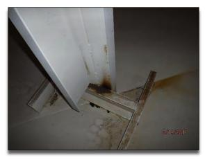
**Photo No. 14** – Interior of R-9A with minor corrosion at seams.
