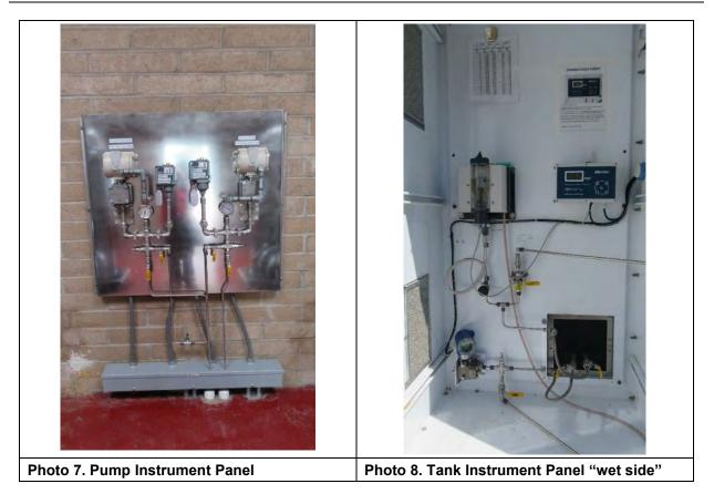
The R16 tank is monitored by a L2000 PLC with small form factor LED Operator Interface. The PLC is provided with battery backup with battery charger in the event of power failure.
