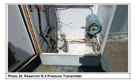
The Reservoir R-3 tank is monitored by a L2000 PLC with small form factor LED Operator Interface. The PLC is provided with battery backup with battery charger in the event of power failure.
