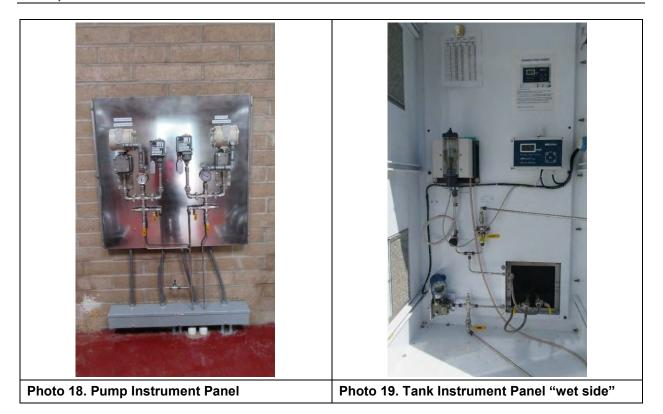
The R16 tank is monitored by a L2000 PLC with small form factor LED Operator Interface. The PLC is provided with battery backup with battery charger in the event of power failure.
