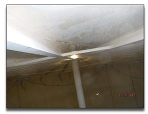
**Photo No. 8** – Interior roof view of R-17 with minor corrosion on roof seams.
