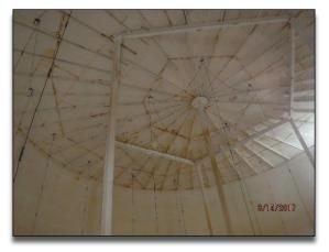
**Photo No. 13** – Interior of R-9A with anodes still suspended from roof.
