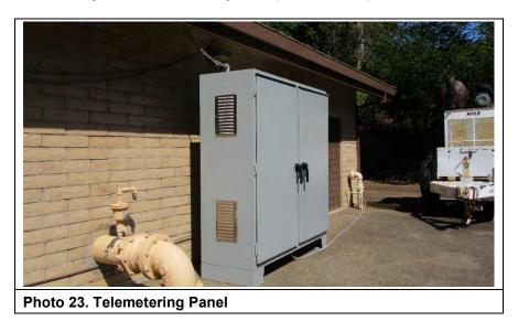
There are three older panels and pedestals containing the instrumentation and communication for Reservoir R-3 tank. Most of the panels are being used as pull boxes between equipment. There is a pressure transmitter in the larger panel (see Photos 24 and 25).
