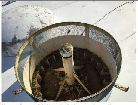
Photo 4-1. Reservoir R-17 Center Vent (with vent hood removed)
