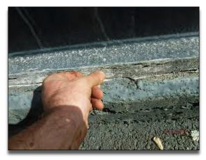
**Photo No. 17** – R-9A annular ring with sealant between annular space and concrete pad.
