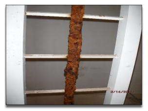
**Photo No. 15 –** R-9A with corrosion product on ladder climbing safety system.
