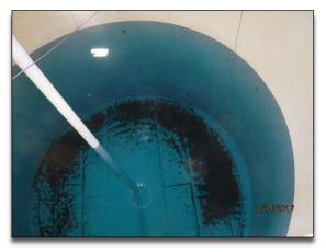
Photo No. 7 - R-17 interior view with debris on bottom.
