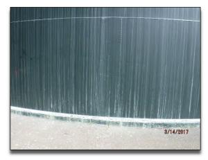
**Photo No. 16** – Exterior of R-9A with chalking present on exterior coating.
