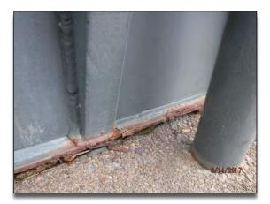
Photo No. 9 – Annular ring of R-17 with corrosion product on ring.
