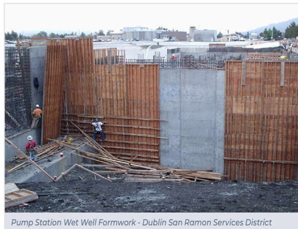
Pump Station Wet Well Formwork - Dublin San Ramon Services District
