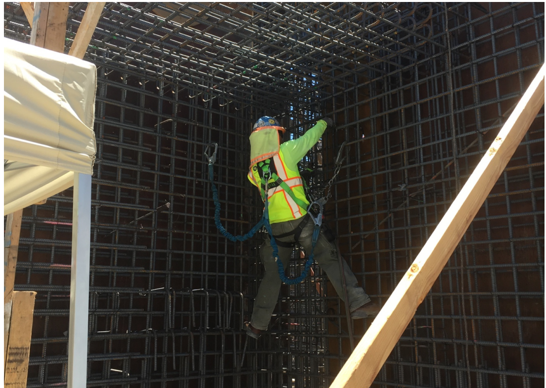
Photograph #2 – Installing Rebar for the new Ballasted Flocculation Structure
