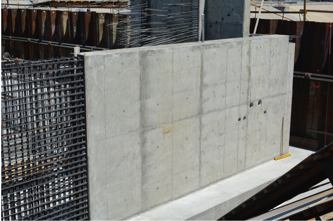
Photograph #1 – Wall Pour #1, Southwest Corner of the Ballasted Flocculation Structure
