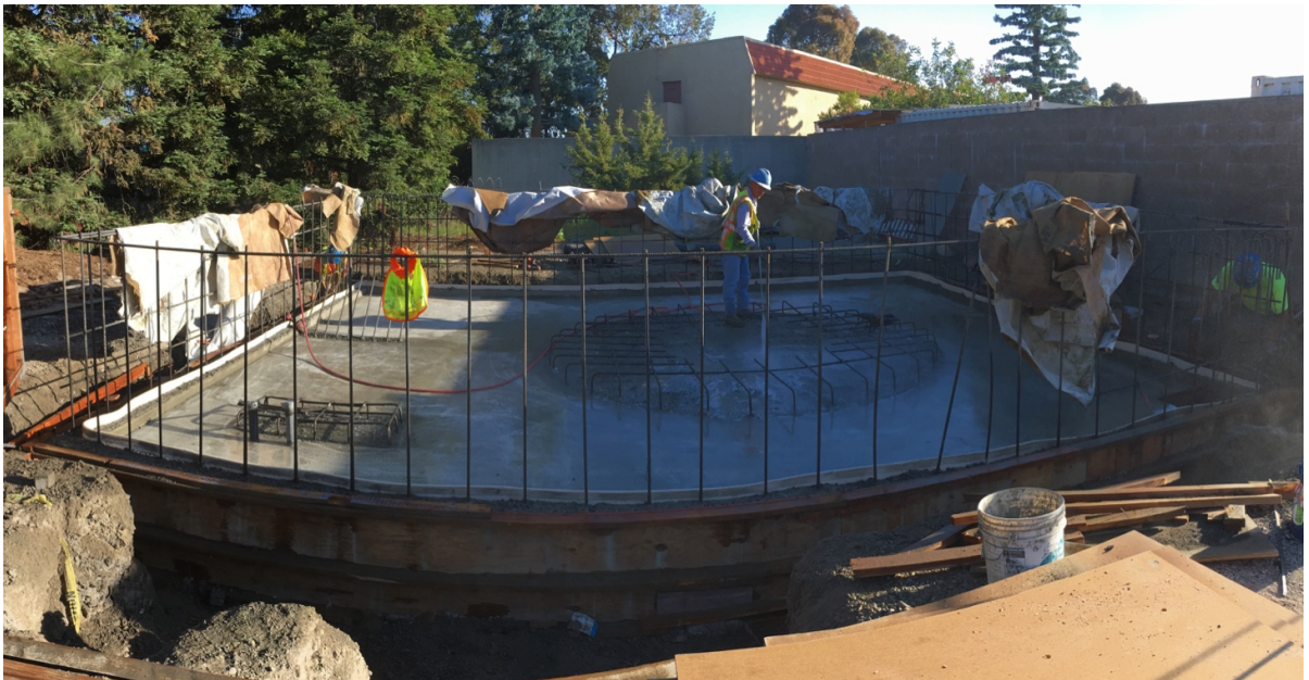
Photograph #4 – Placing new Coagulant Area Base Slab Concrete
