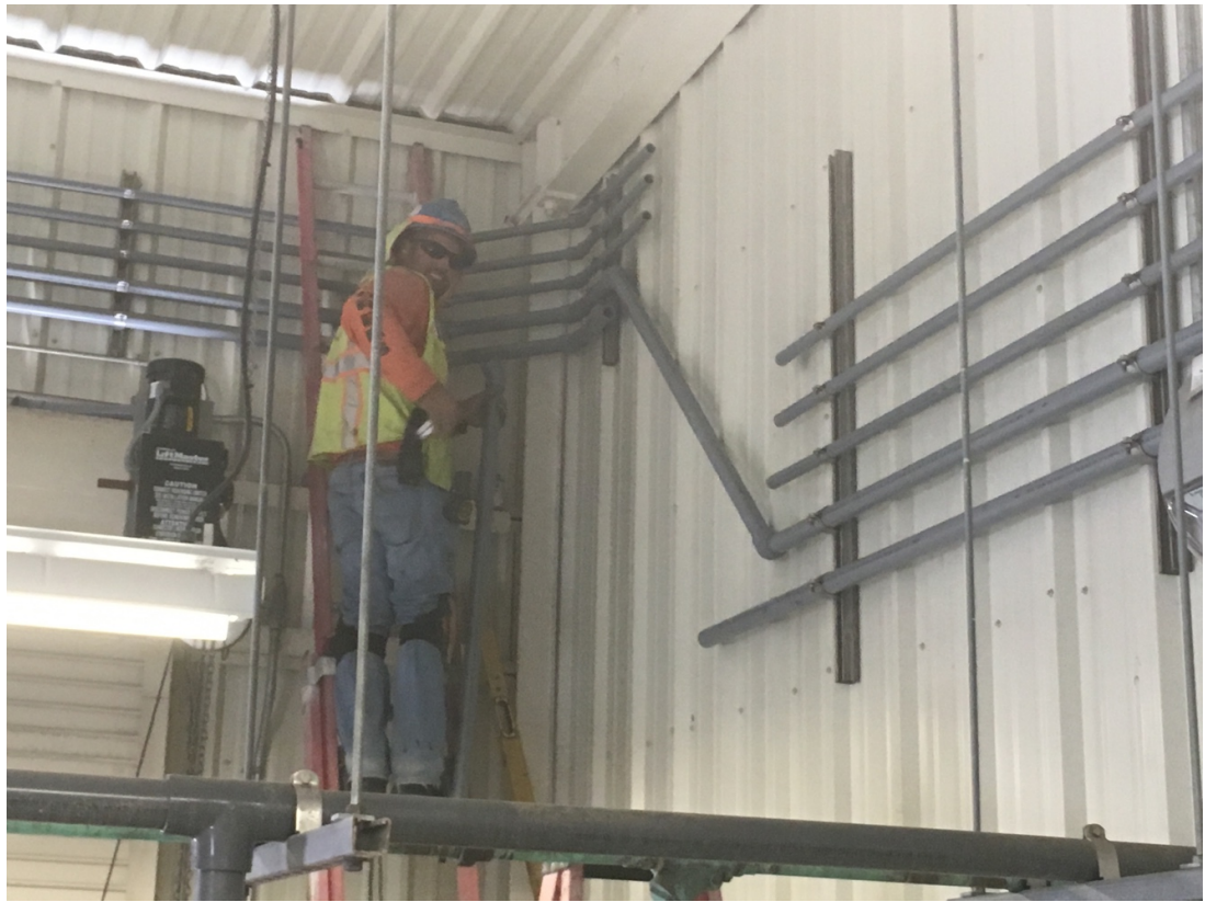
Photograph #3 – Installing new Chemical Piping in Building O
