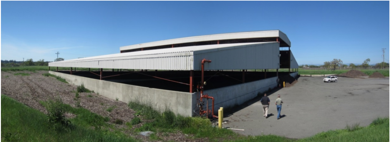
Figure 2-7: Alpha Farm Biosolids Storage Building
