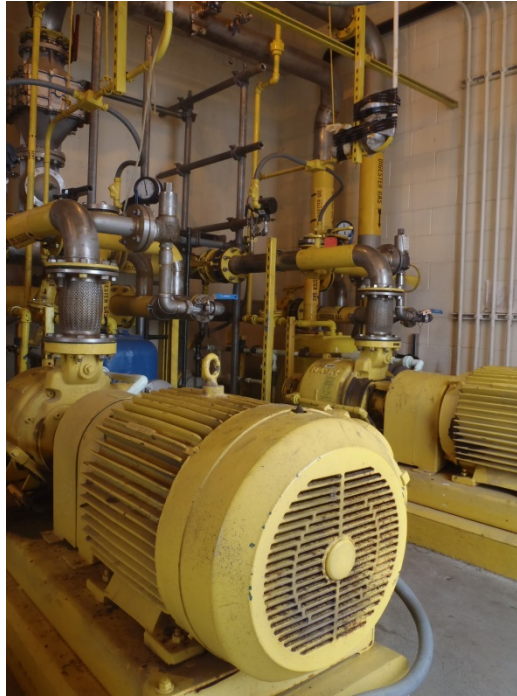
Figure 1-10: Digester Gas Mixing Pumps
