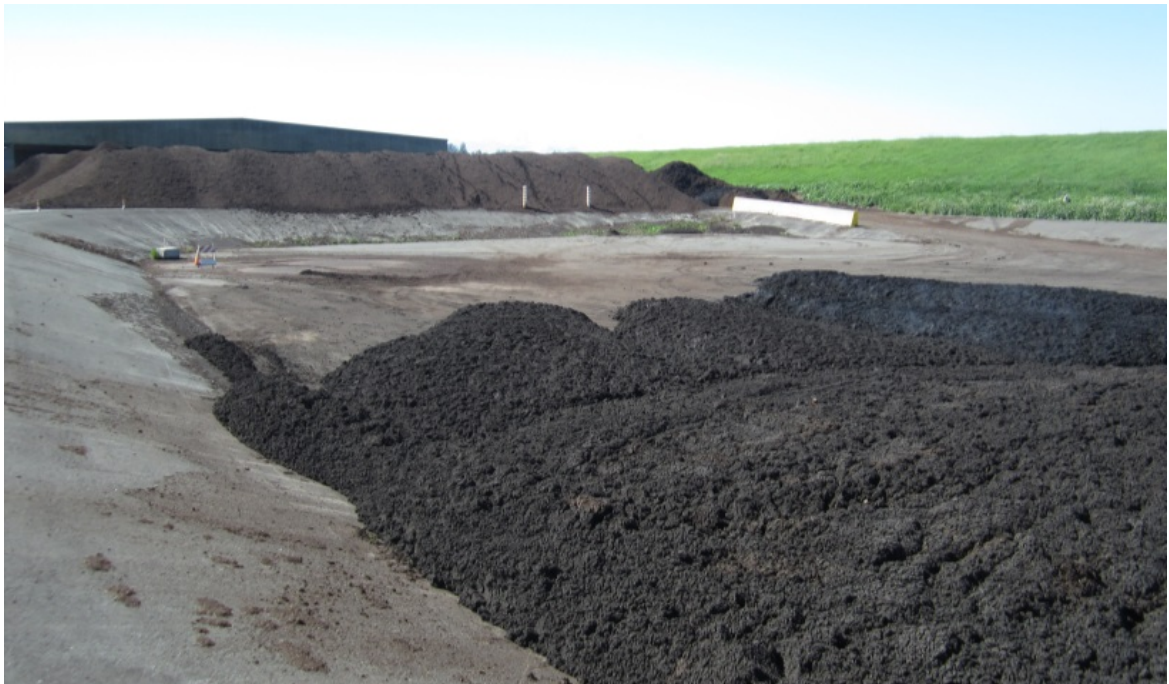
Figure 2-6: Composting Facility Pond Biosolids Storage Area
