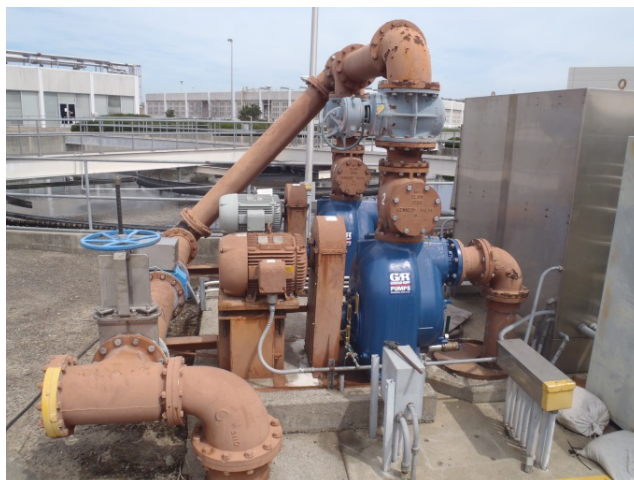
Figure 1-9: RAS Pumps Adjacent to the Clarifier
