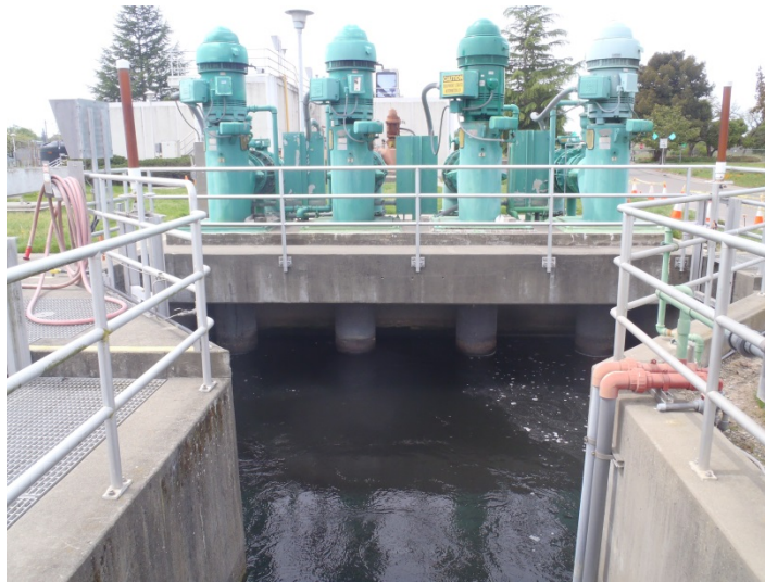
Figure 1-3: Tertiary Filter Wet Well Pumps
