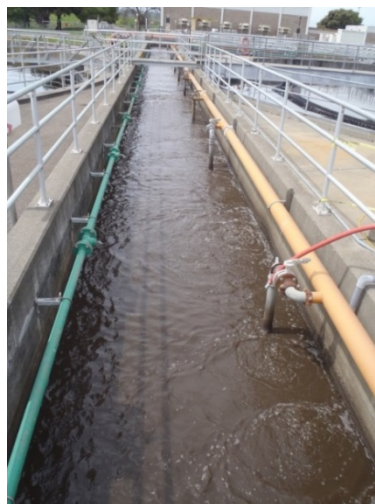
Figure 1-7: Mixed Liquor Channel with Aeration
