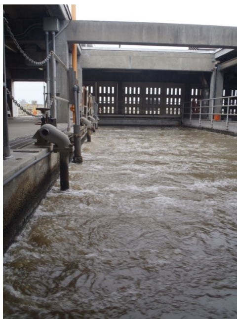
Figure 1-11: Grit Tank with Aeration
