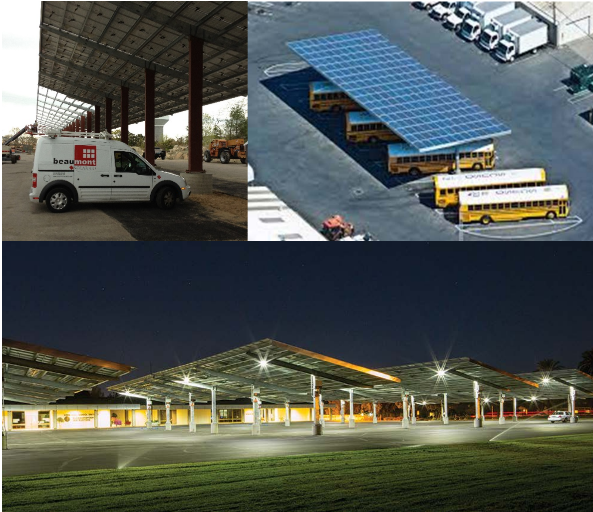
Figure 7-3: Example Solar PV Carport Structures
