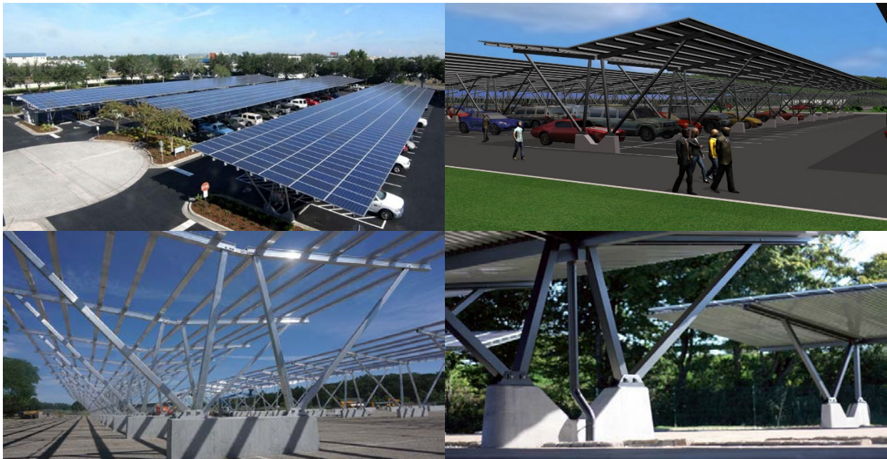
Figure 7-2: Example Solar PV Carport Structures
