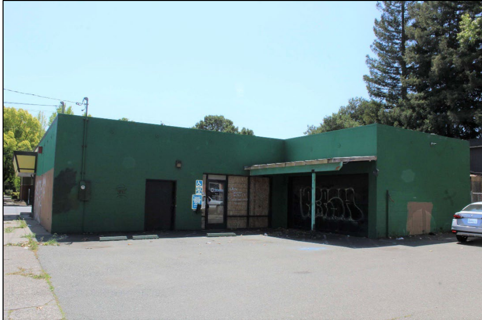
Photo 18: Building at 353 College, looking SW
