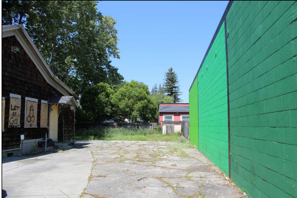
Photo 14: Side yard, looking north
