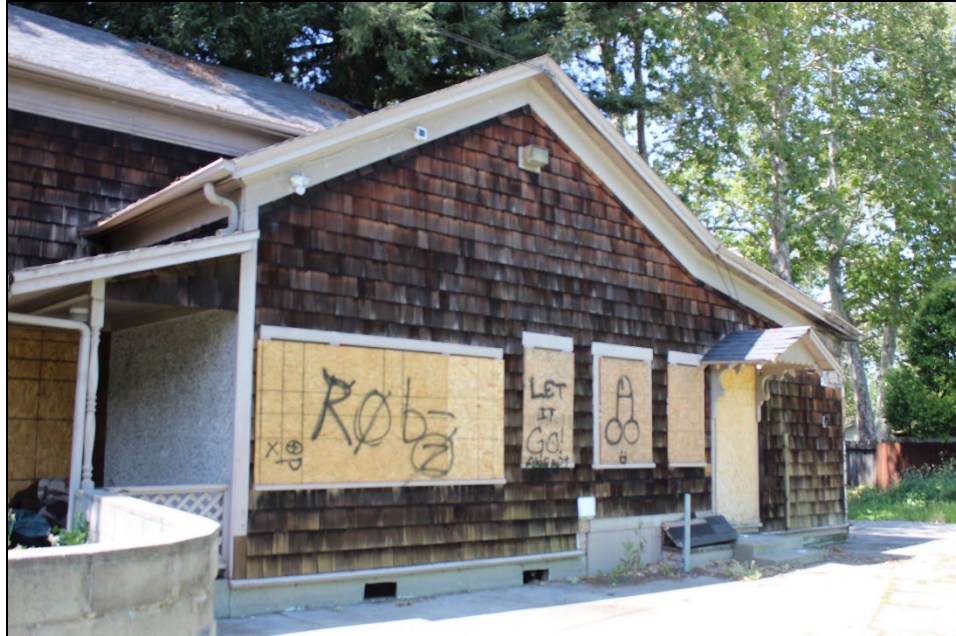
Photo 5: East side façade, looking NW
