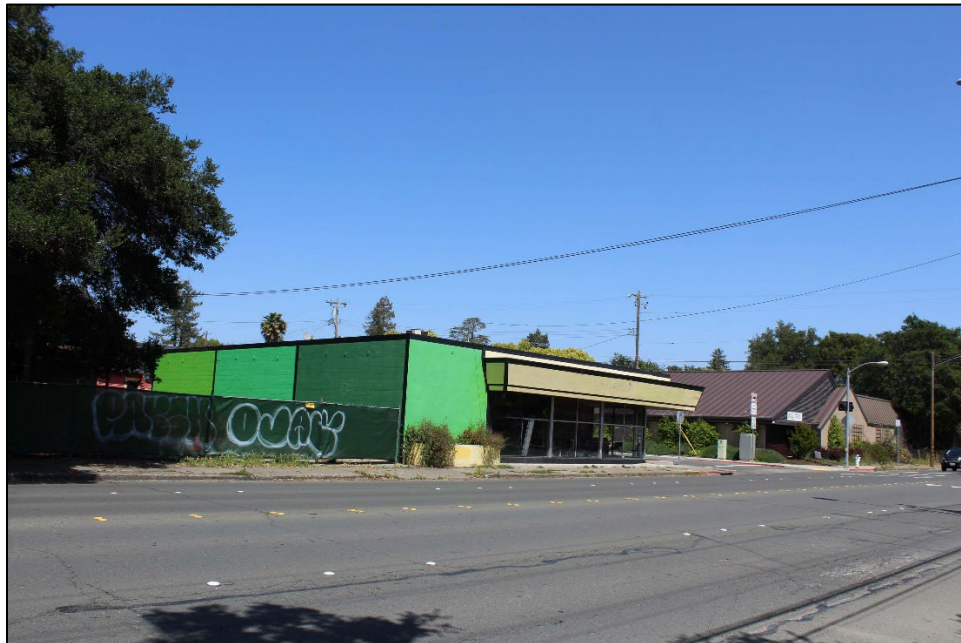
Photo 17: Building at 353 College, looking NE
