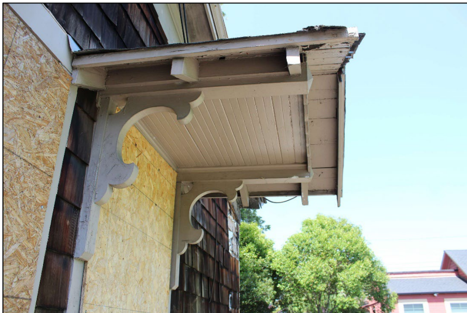
Photo 6: Gable detail, east side facade
