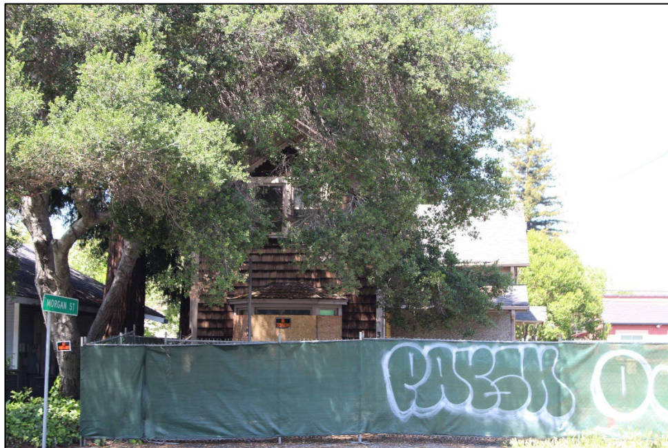
Photo 2: North (front) façade
