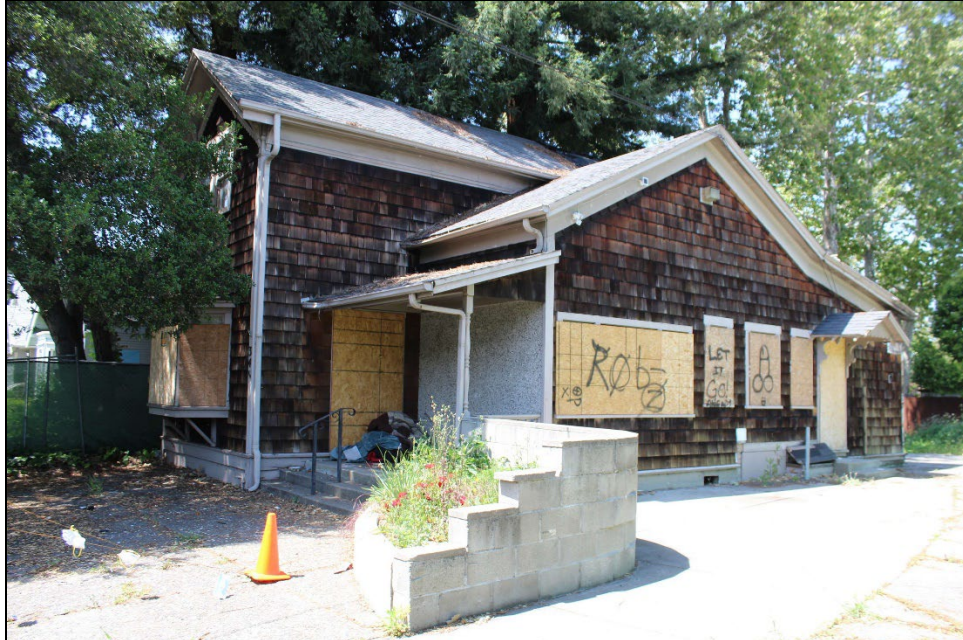
Photo 1: North (front) and east side facade
