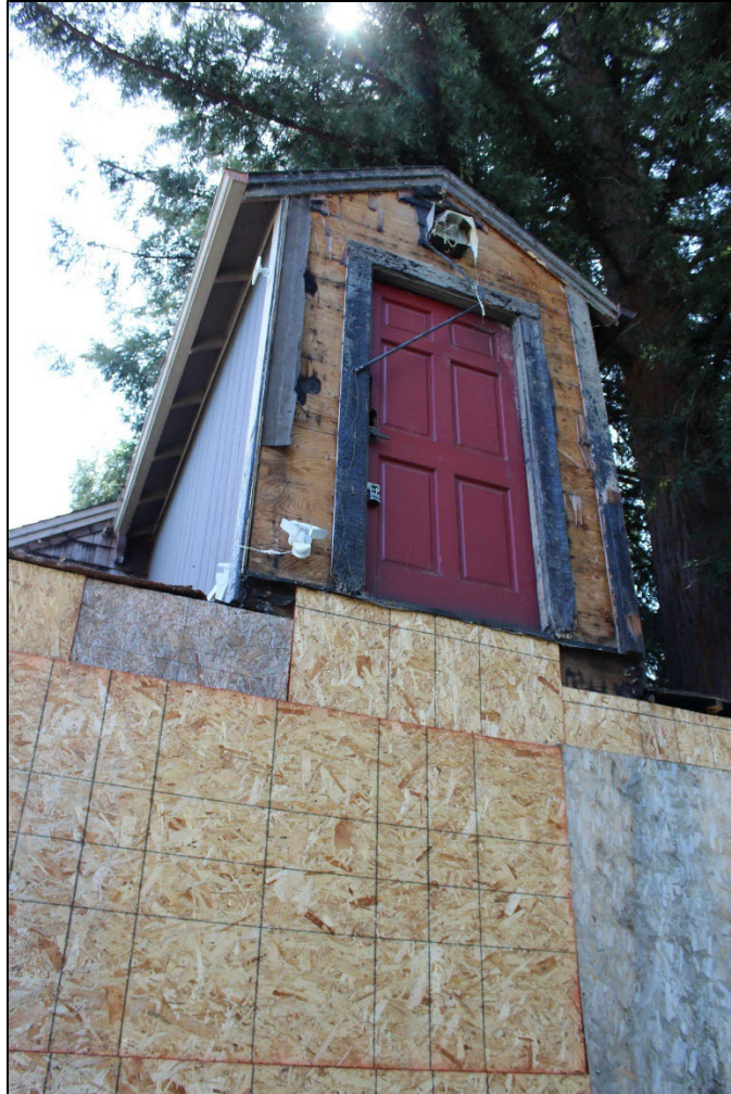
Photo 7: Enclosed hallway and entry door, north façade, second floor
