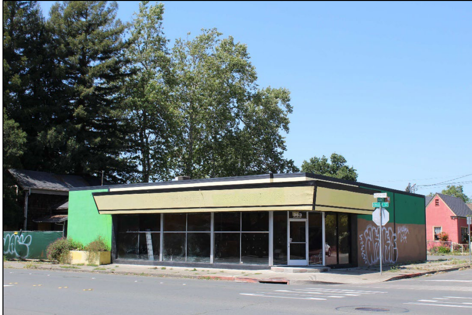
Photo 16: Building at 353 College, looking NW
