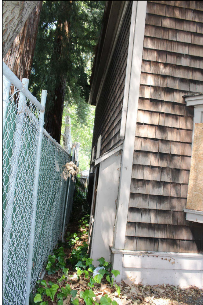
Photo 9: West side façade, looking north
