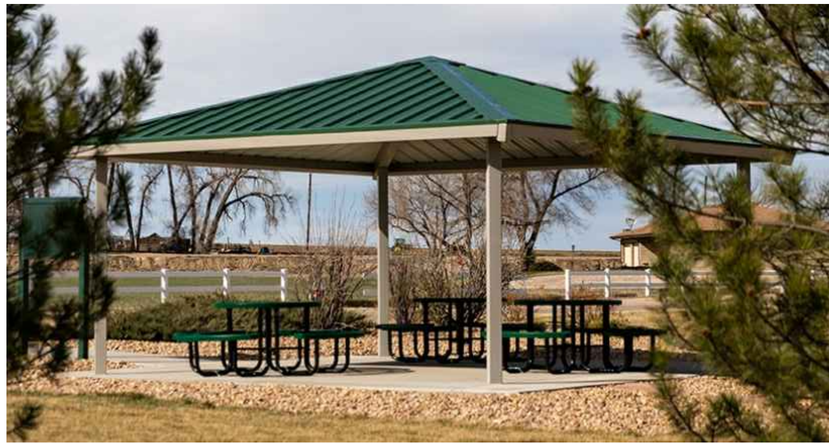
OVERHEAD SHADE STRUCTURE
