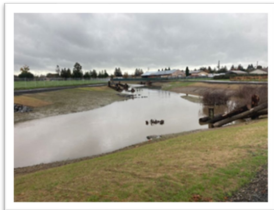
Figure 21 - Lower Colgan Creek Phase 2 after initial channel restoration, 2021
