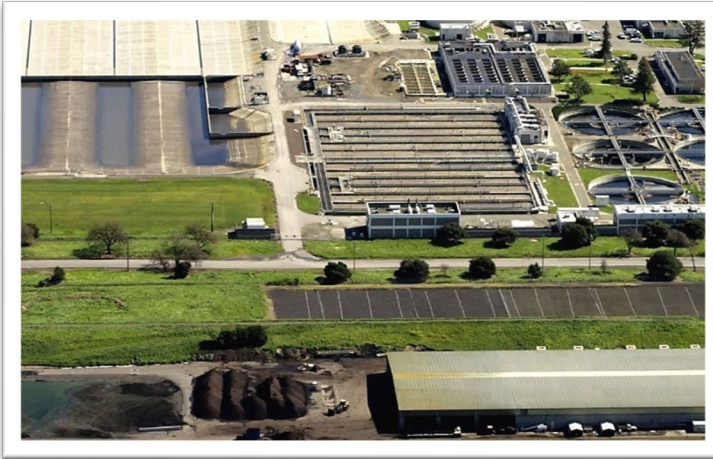
Figure 18 - Laguna Treatment Plant
