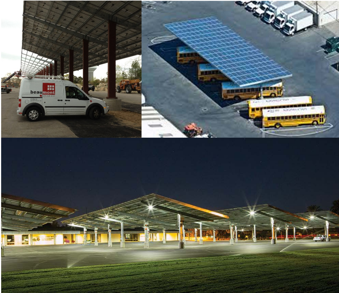
Figure 7-3: Example Solar PV Carport Structures
