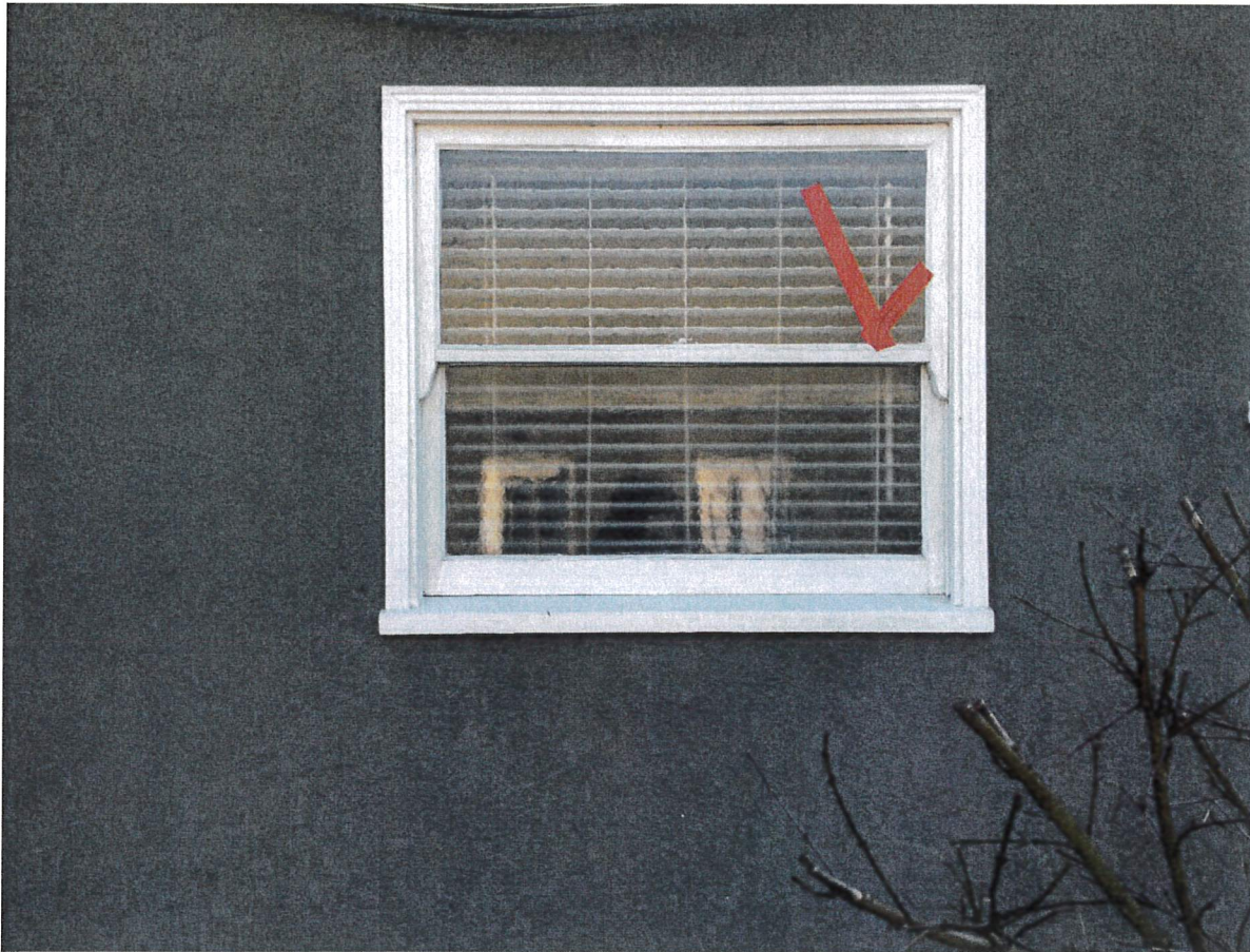
Window 4 – Bathroom window
