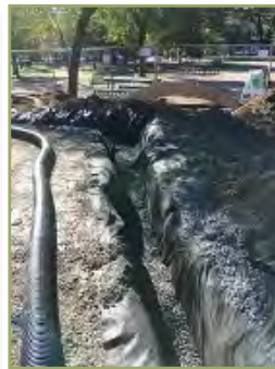
Drainage Installation.
