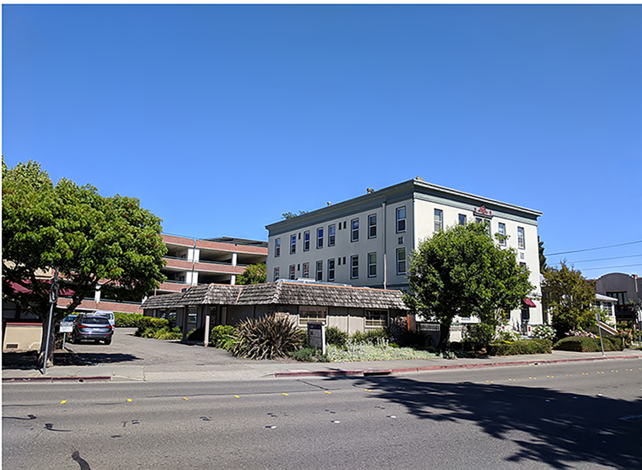
VIEW FROM B STREET
