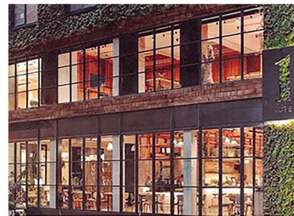
4 STEEL SASH STOREFRONT WINDOWS
