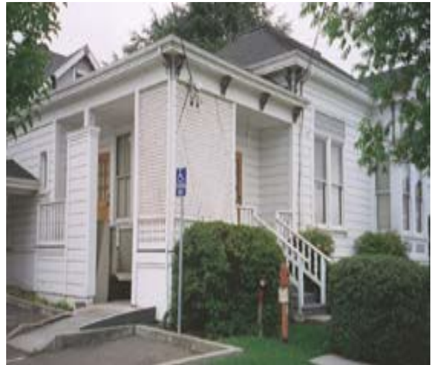
Mechanical lift is screened by lattice work on this Queen Anne house used as an office.
