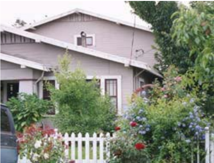
A second-story addition to this St. Rose Bungalow has been set back from the existing building front.
