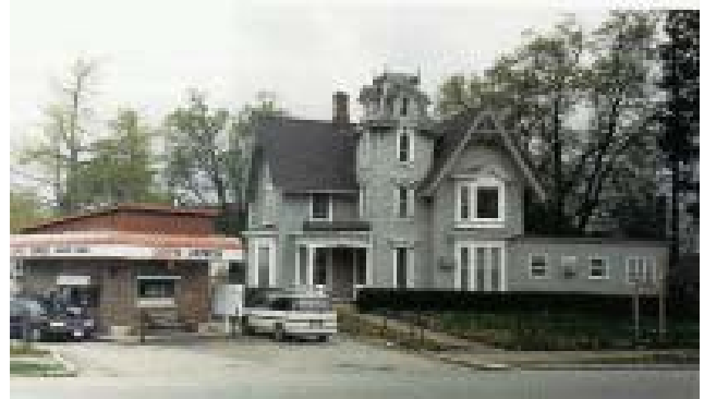
Insensitive new construction, along with an inappropriate addition, has compromised the integrity of this Gothic Revival Style house.
