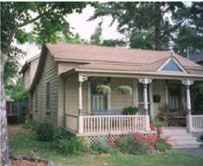
A two-story addition has been placed inconspicuously To the rear of this one-story Queen Anne Cottage.
