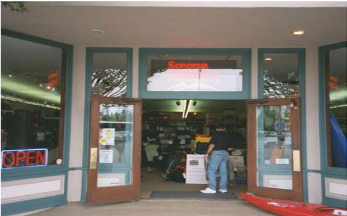
New storefront in the Railroad Square Preservation District “reads” as a traditional storefront.
