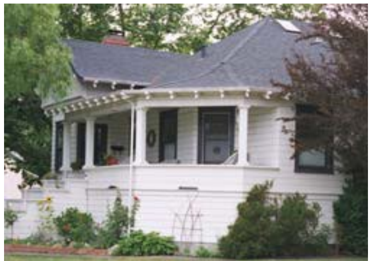
A porch is one of the main defining features of a house and should not be enclosed or removed.
