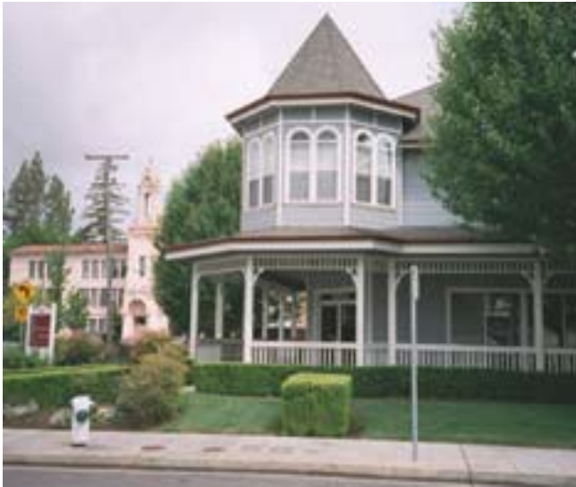
New construction in the St. Rose Preservation District provides both office use (first floor) and residential units (second floor).
