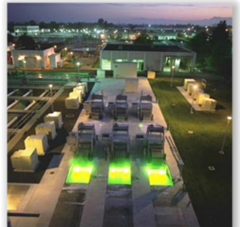
Laguna Treatment Plant
