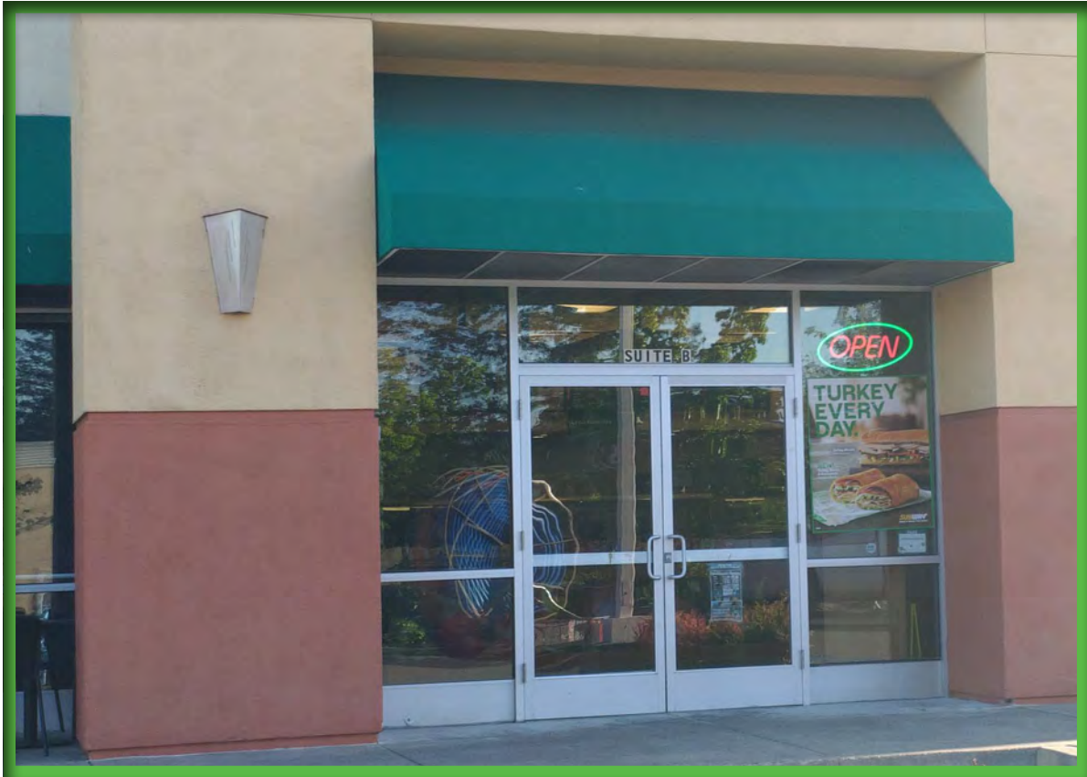
G. Left side of adjacent property - Subway.
