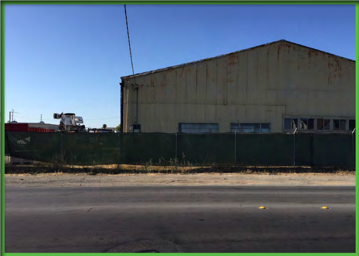
D. Adjacent North Property
