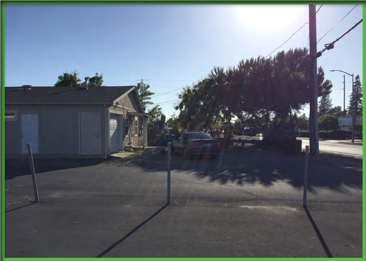
A. East Front Facade To Be Improved with ADA Ramp and Landscaping
