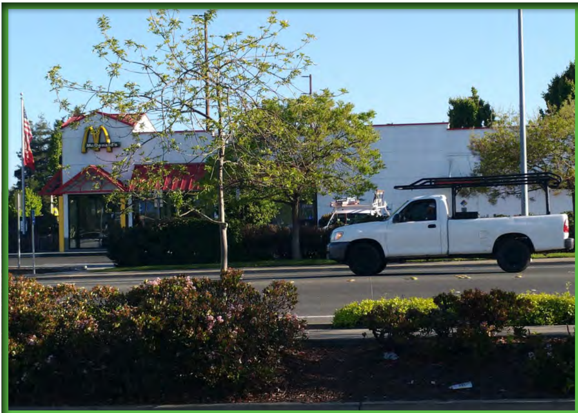
G. Neighboring property - McDonald's on Santa Rosa Ave
