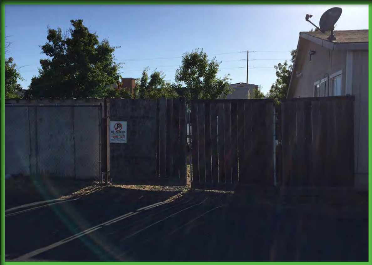
I. Dilapidated Rear Gate and Fence to be Removed
