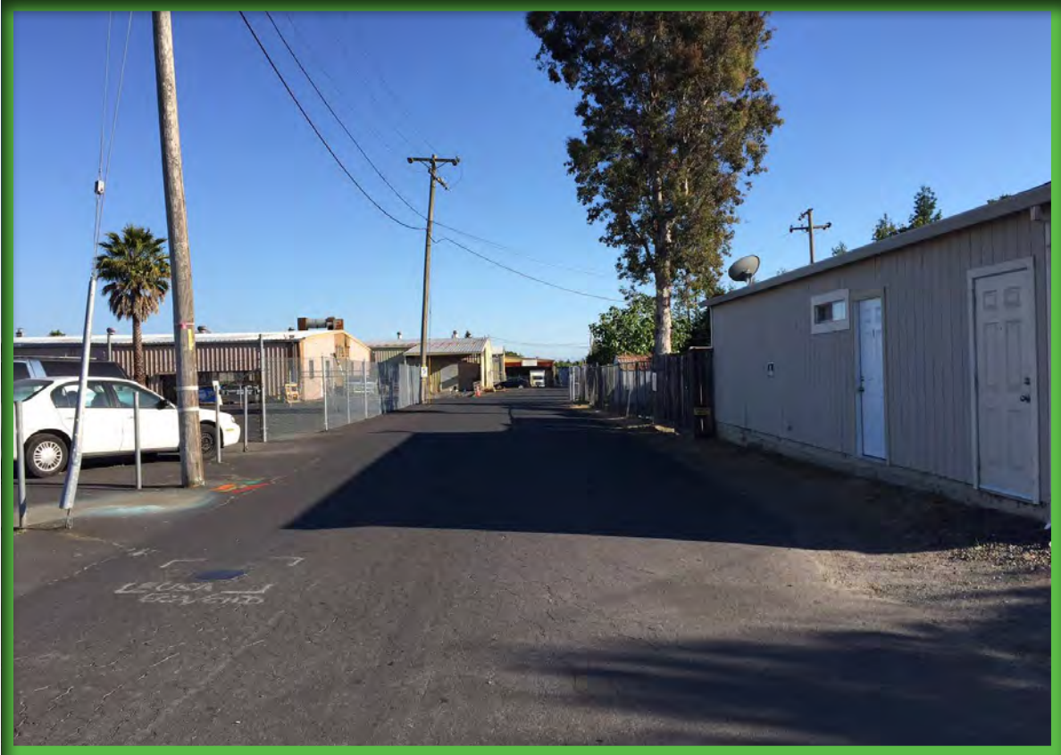
C. Side (East) Facade with Driveway & Access Doors. Will be cleaned and maintained for visitors.
