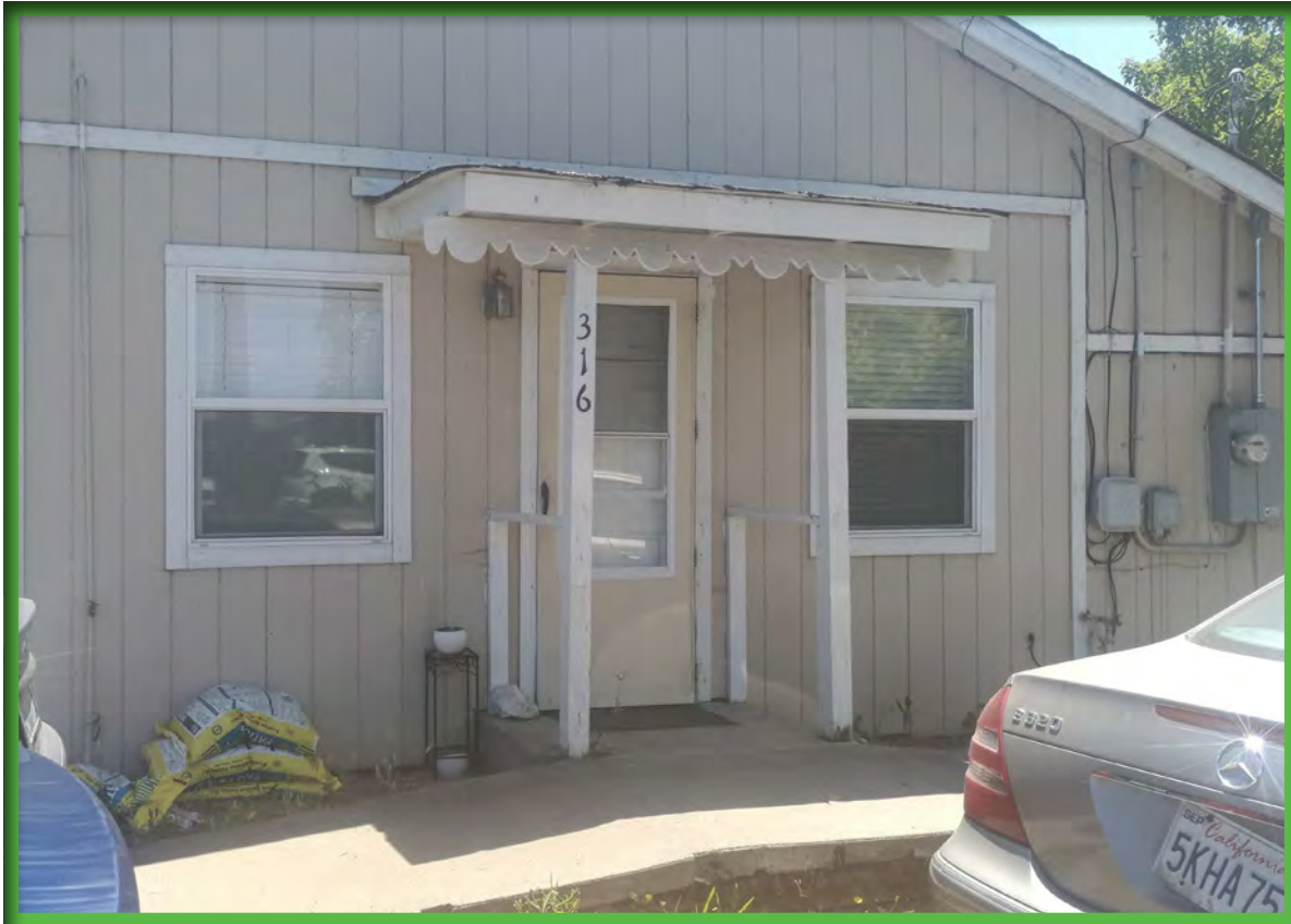
G. Front Entry to Be Improved with an Attractive Ramp, Railing, Parking Area, and Landscaping.
