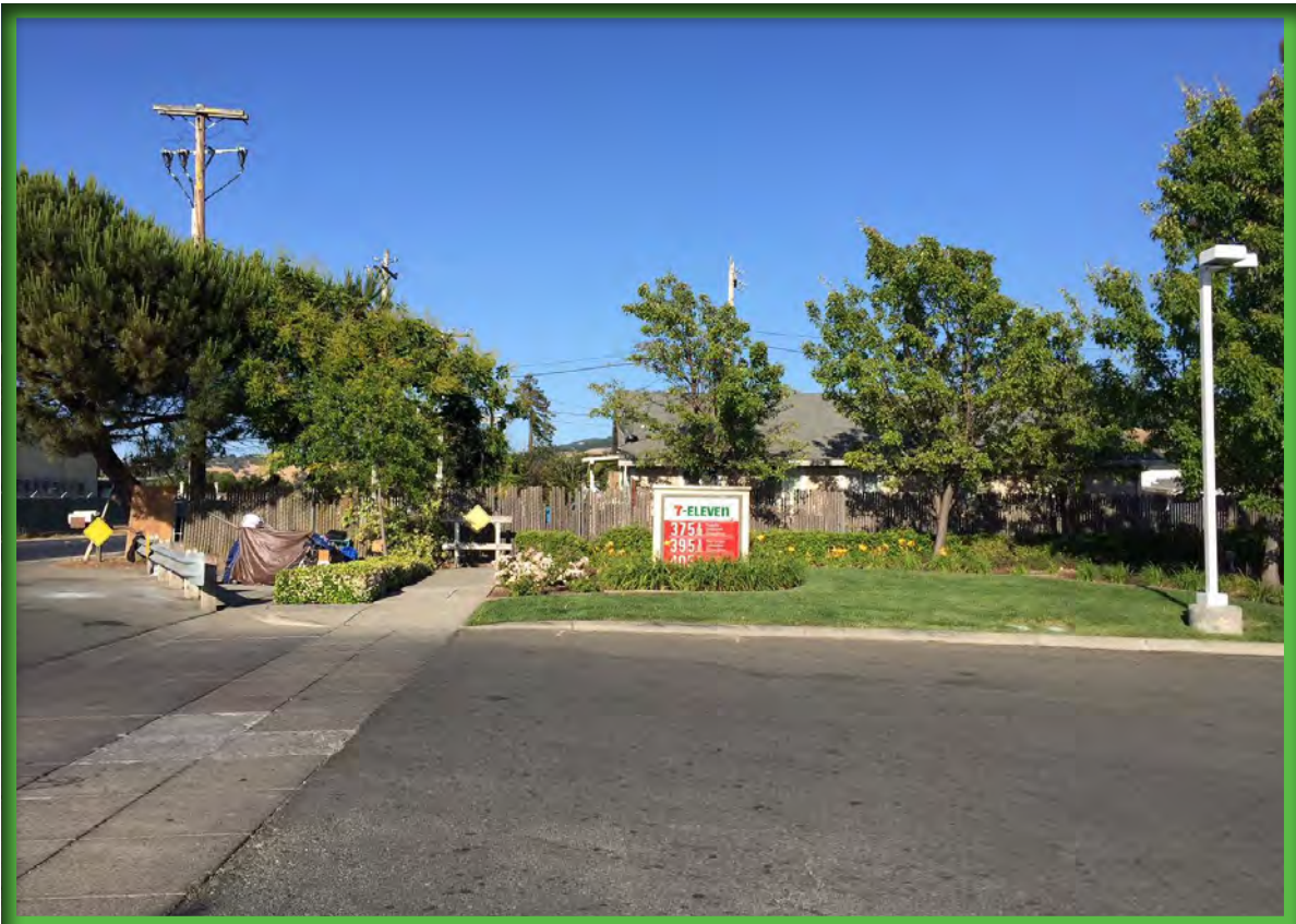
B. West Front Facade To Be Improved
