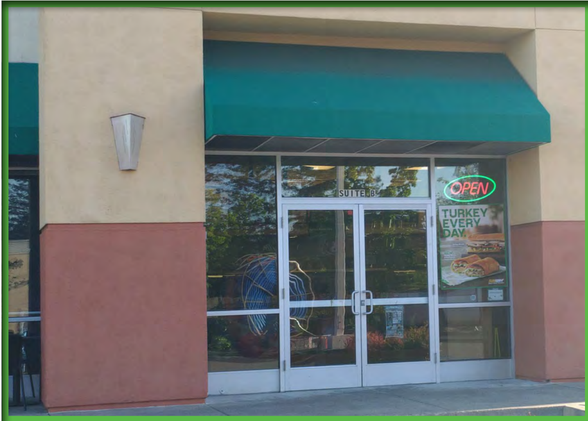
G. Left side of adjacent property - Subway.
