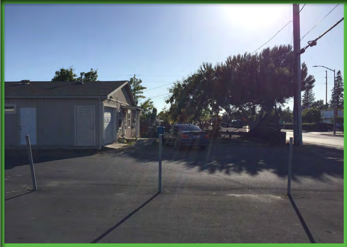
A. East Front Facade To Be Improved with ADA Ramp and Landscaping
