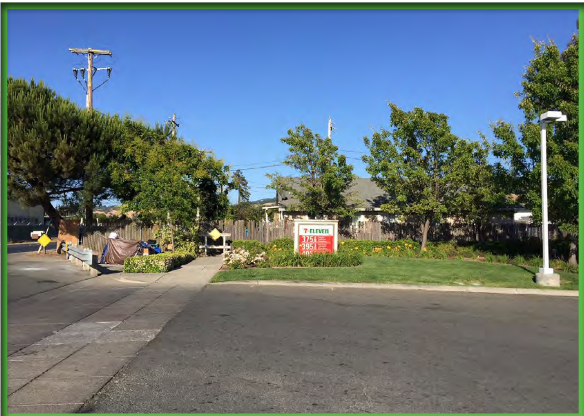
B. West Front Facade To Be Improved
