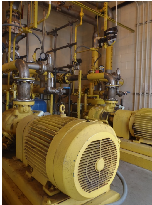
Figure 1-10: Digester Gas Mixing Pumps
