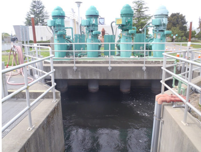
Figure 1-3: Tertiary Filter Wet Well Pumps
