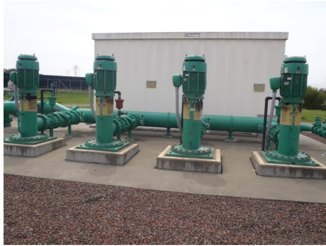
Figure 1-6: Recycled Water (3W) Booster Pumps
