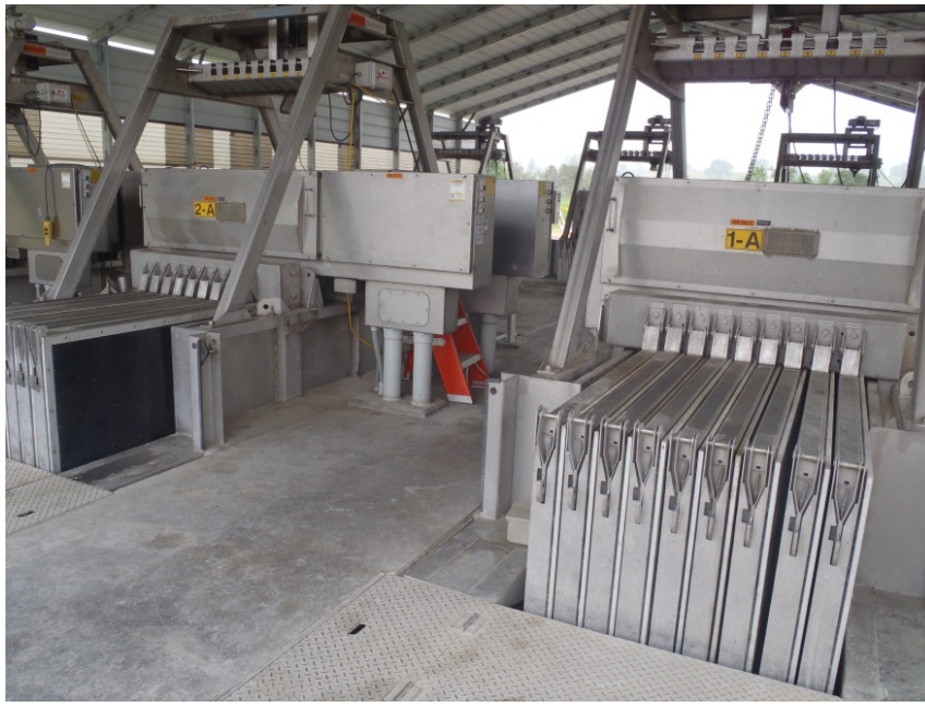
Figure 1-4: UV Disinfection Equipment
