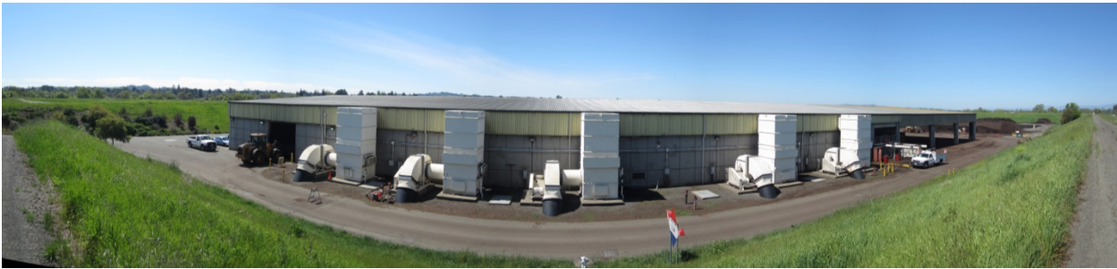
Figure 2-1: Panorama View of the Laguna Subregional Compost Facility
