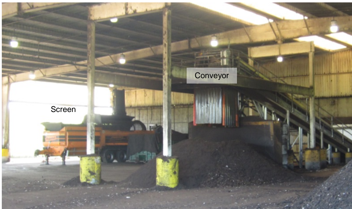
Figure 2-5: Screening Equipment Location Relative to Conveyor
