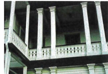
Decorative wood exterior or interior features should not be cleaned abrasively. Photo: NPS files.
