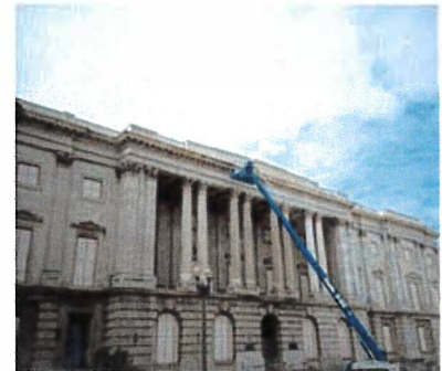
Low-to-medium-pressure steam (hot-pressurized water washing) is a gentle method of softening heavy soiling deposits and cleaning historic marble. Photo: NPS files.
