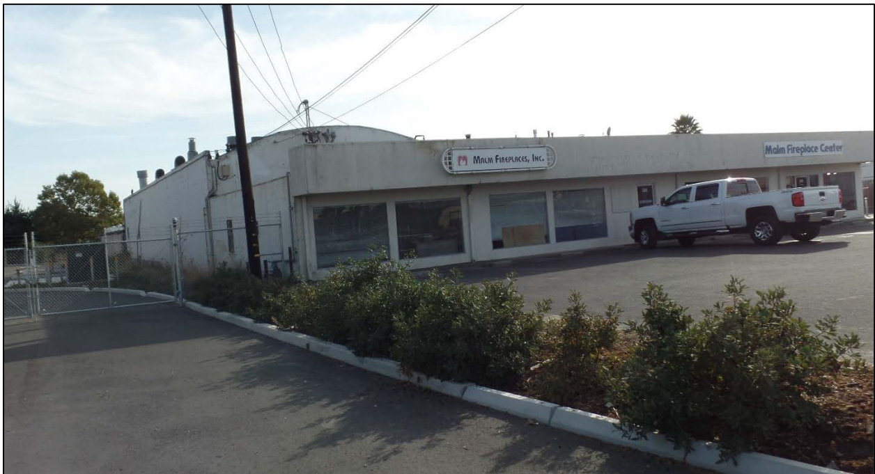
368 Yolanda Avenue, view to southwest. Note barrel roof shape.
