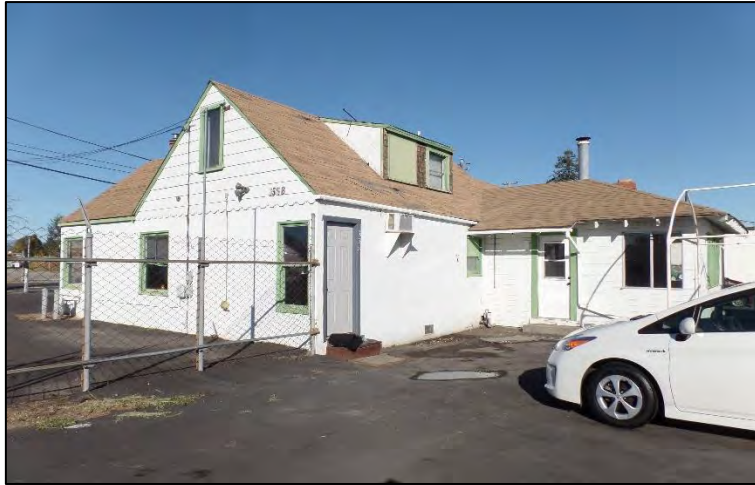
350/358 Yolanda Avenue west and south façades, view to northeast
