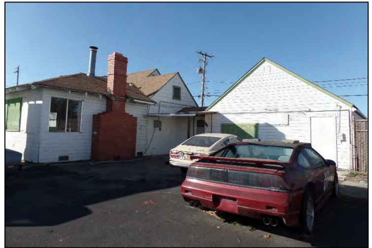
350/358 Yolanda Avenue east and south façades, view to northwest.
