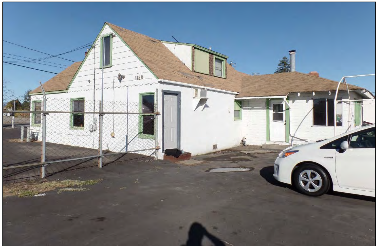
350-358 Yolanda Avenue, view to northeast
