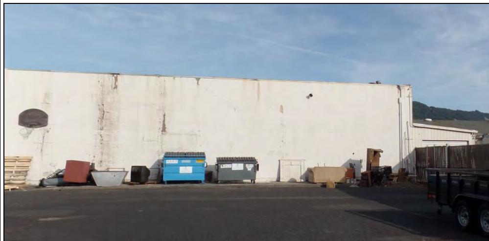
368 Yolanda Avenue south end of west façade, view to east.
