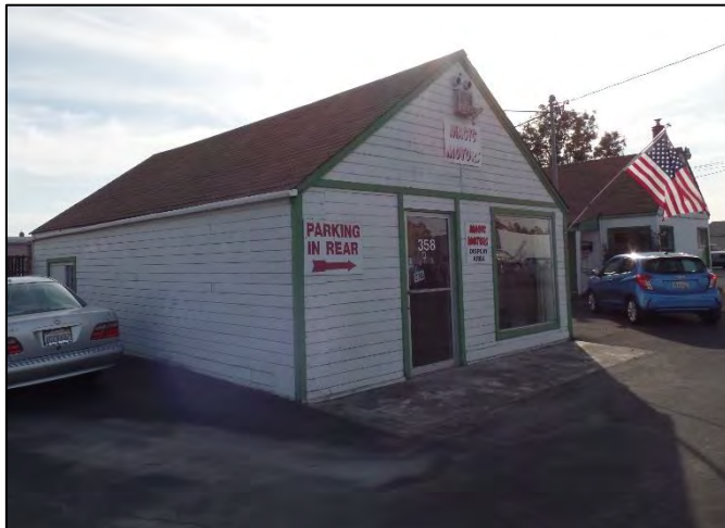
350/358 Yolanda Avenue former garage/barn east and south façades, view to southwest.
