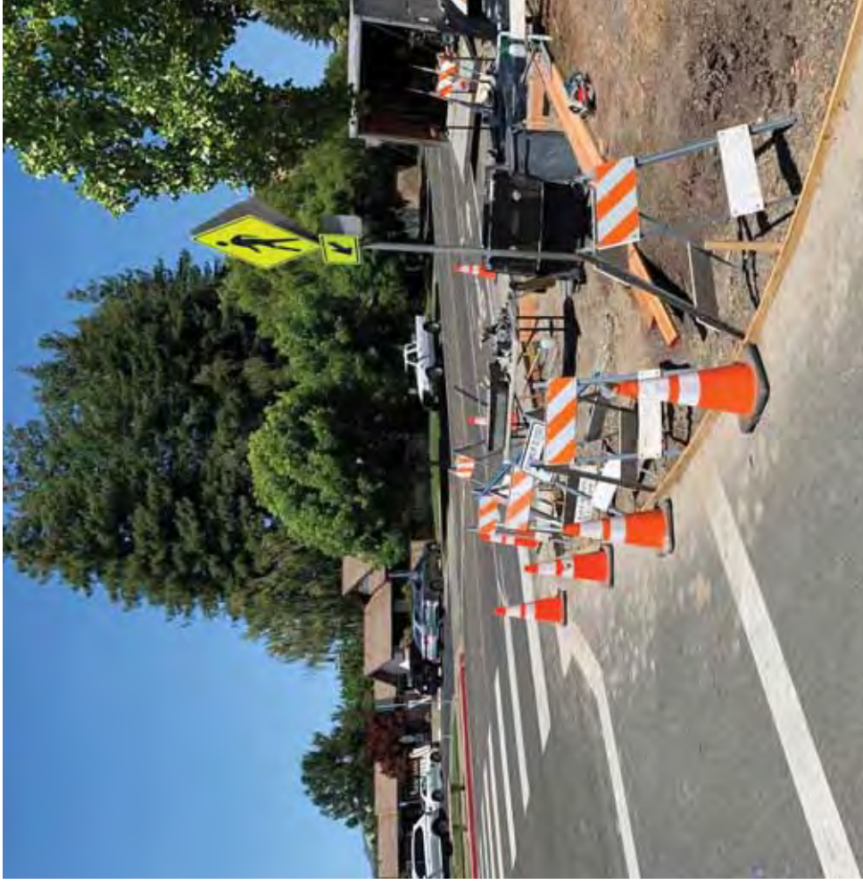
Construction of a new curb and ramp to support a new Rectangular Rapid Flashing Beacon in Santa Rosa, CA.
