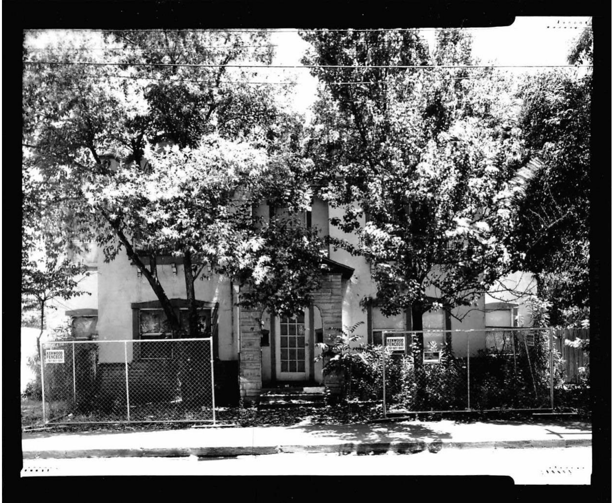
608 Morgan Street - Photo #1 - EXTERIOR, OVERVIEW OF PRIMARY (WEST) FACADE, VIEW TO NORTHEAST.
