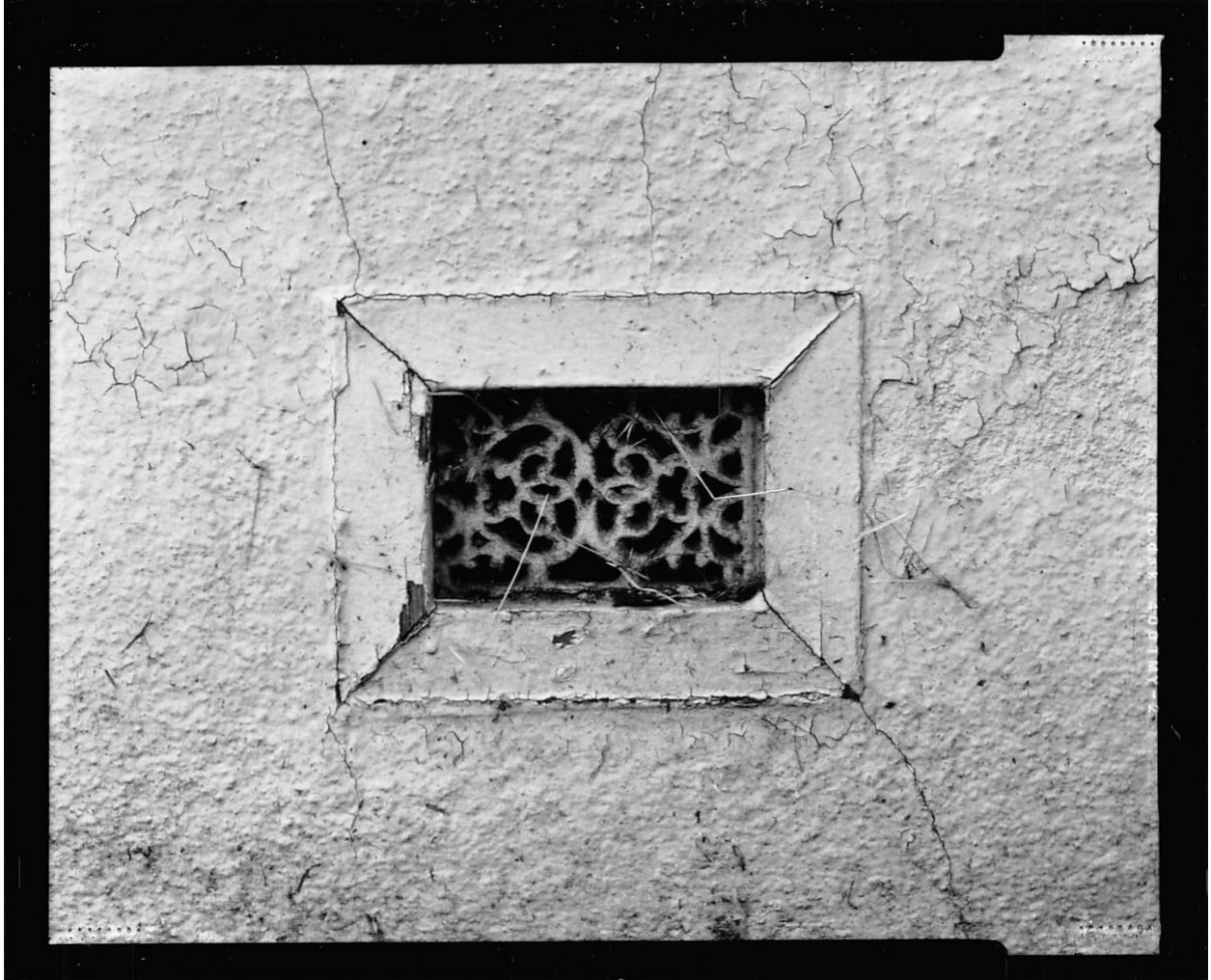
608 Morgan Street - Photo #8 - EXTERIOR, DETAIL OF VENT, VIEW TO THE SOUTHEAST.
