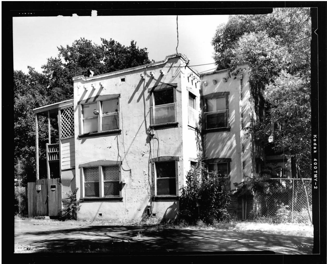
608 Morgan Street - Photo #4 - EXTERIOR, OVERVIEW OF SECONDARY (NORTH) FACADE, VIEW TO SOUTHEAST.
