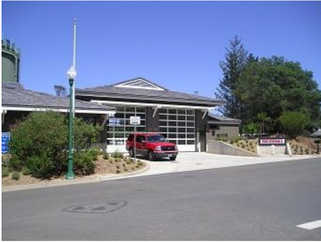
Figure 27: Santa Rosa Fire Department Station 5 (New Station) 2201 Newgate Court
