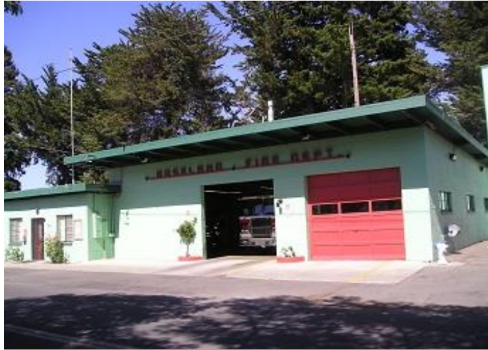
Figure 30: Santa Rosa Fire Department Station 8 830 Burbank Avenue
