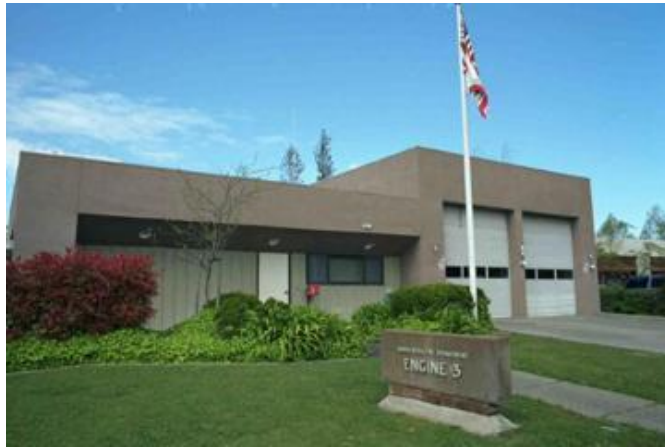
Figure 24: Santa Rosa Fire Department Station 3 3311 Coffey Lane
