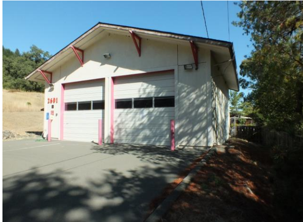
Figure 36: Rincon Valley Fire Protection District Station 25 2601 Calistoga Road
