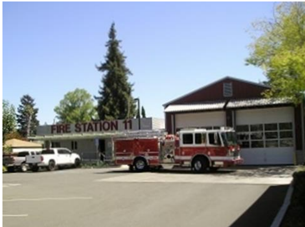
Figure 32: Santa Rosa Fire Department Station 11 550 Lewis Road
