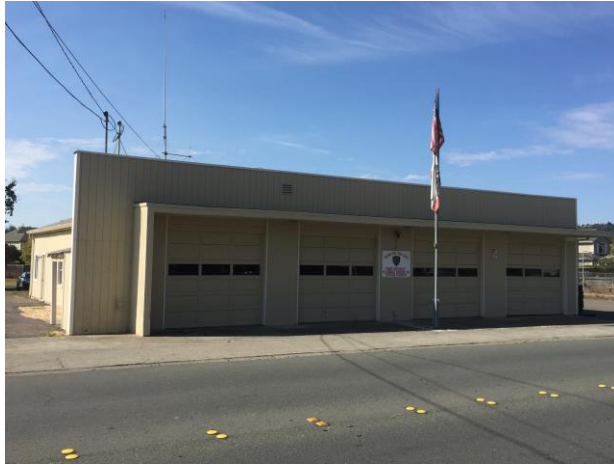
Figure 33: Rincon Valley Fire Protection District Station 20 91 Middle Rincon Road
