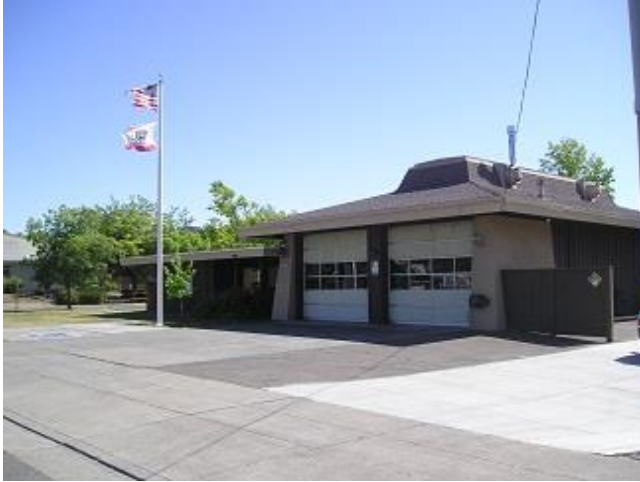
Figure 25: Santa Rosa Fire Department Station 4 1775 Yulupa Avenue
