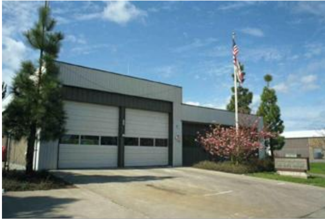
Figure 23: Santa Rosa Fire Department Station 2 65 Stony Point Road
