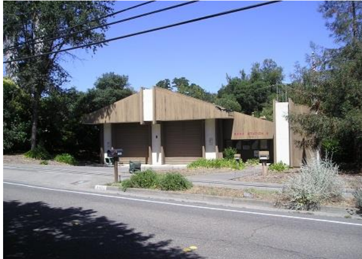
Figure 26: Santa Rosa Fire Department Station 5 (Old Station) 2201 Newgate Court
