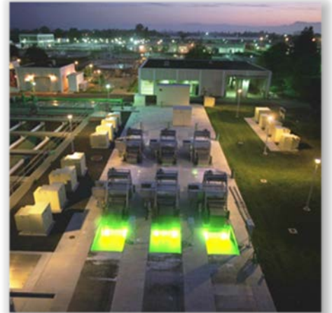
Laguna Treatment Plant
