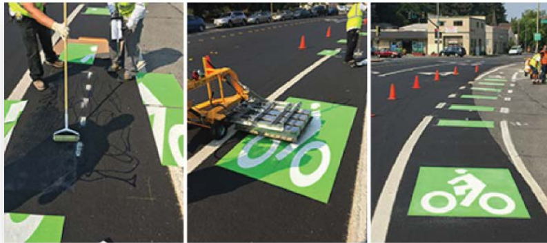
Green bike lane installation on Sonoma Avenue at Santa Rosa Avenue
