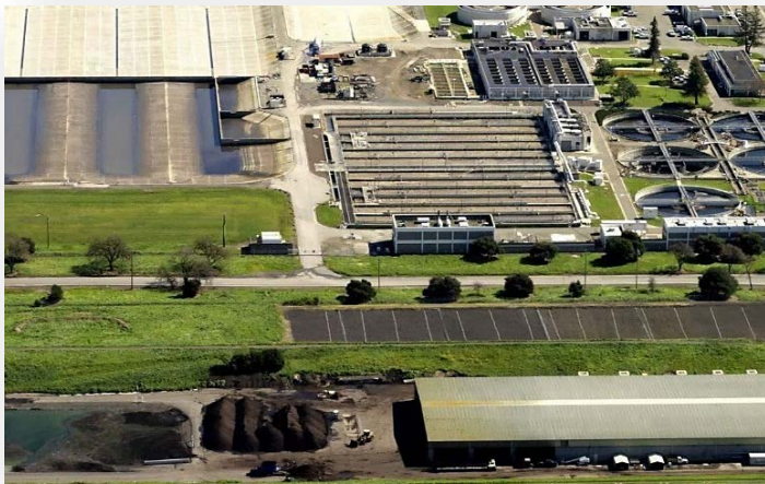
Laguna Treatment Plant
